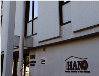
HANO Main Office
