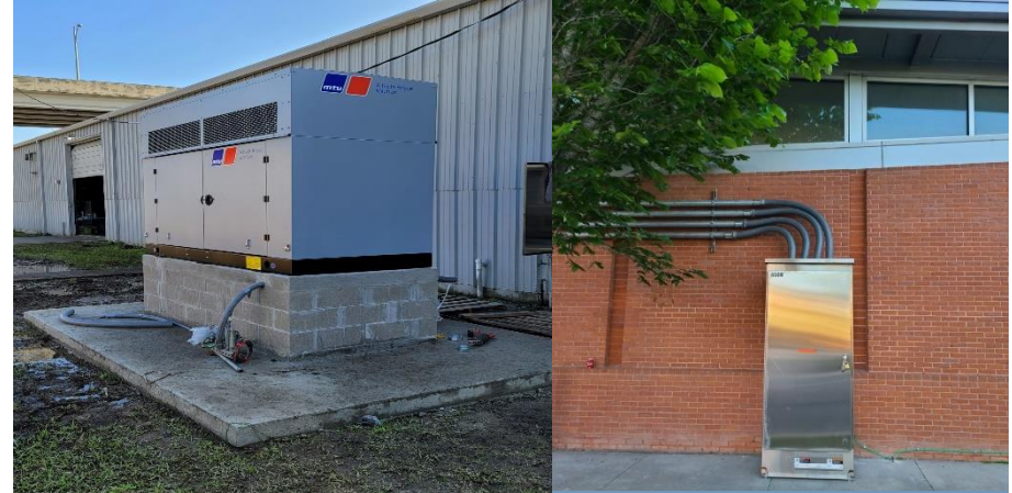
Citywide Generator Installation
