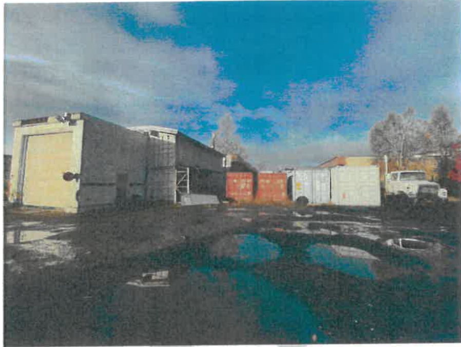
Photograph 4.0-3: Rear Parking/Storage Area
