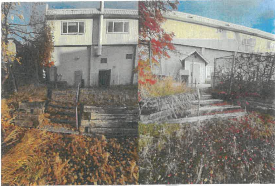
Photograph 8.0-4 & 5: Railroad Tie Steps
