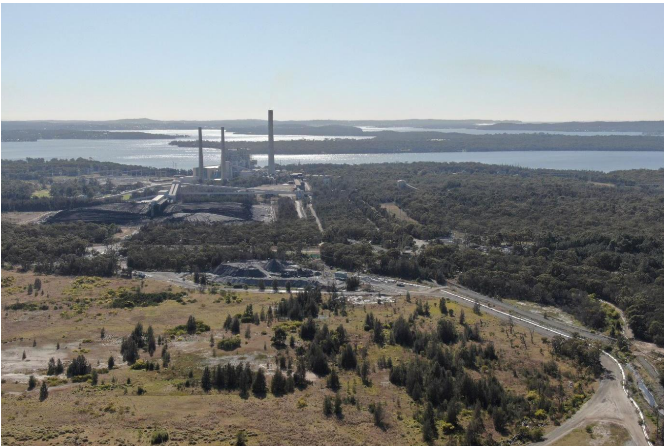
Vales Point power station. HCEC.
