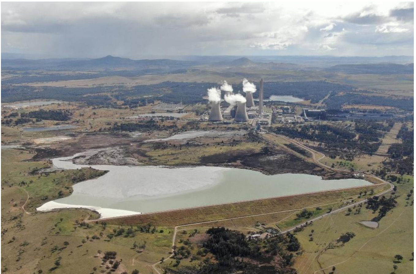
Bayswater power station. HCEC.
