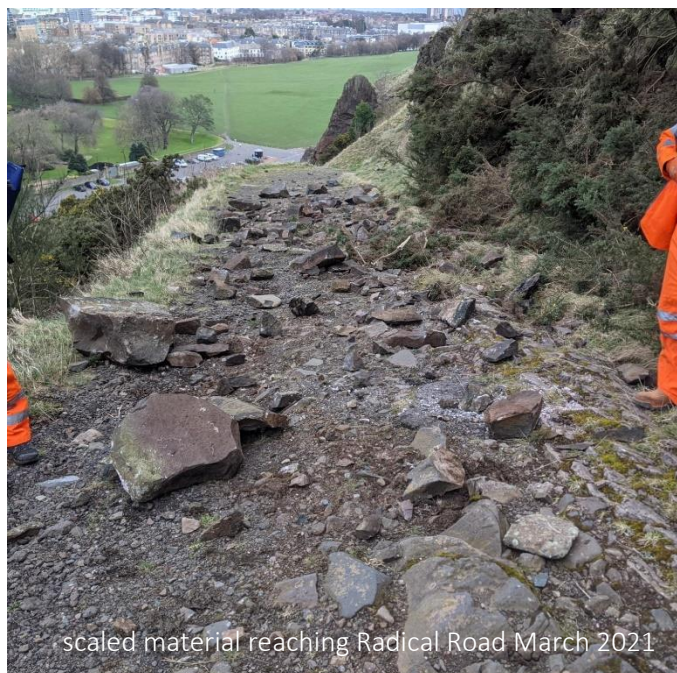
rock scaling Salisbury Crags from ropes March 2021
