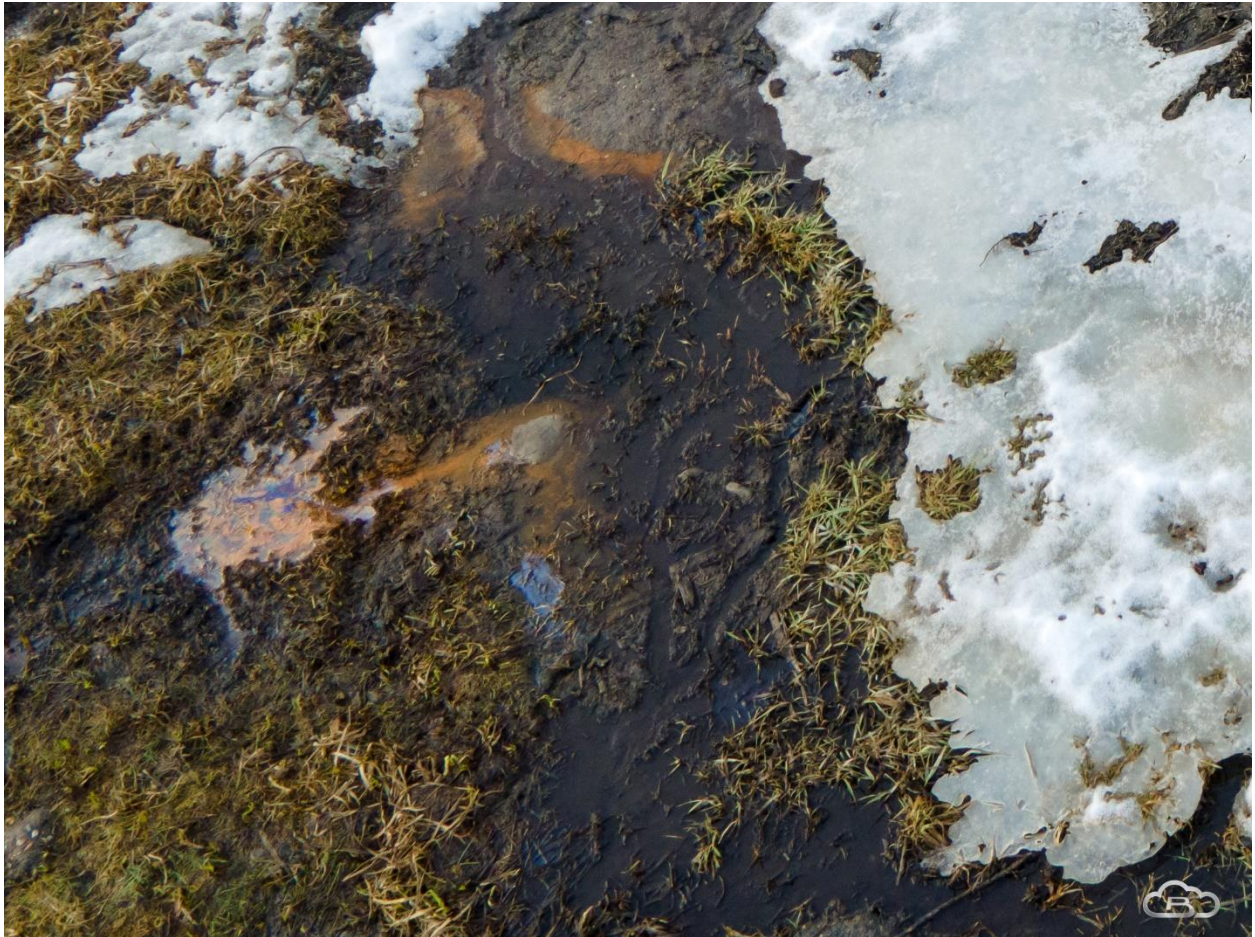
Figure 3. March 2022 Drone Image of Mississippi River Crossing 1 Fracout with drilling muds still leaking to surface wetlands 9 months after river crossing was complete.
