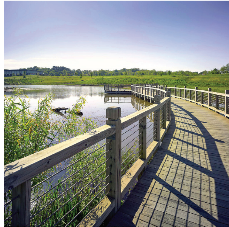
TREATMENT WETLAND WITH BOARDWALK ACCESS
