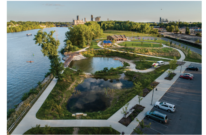
TREATMENT TRAIN CLEANING RUNOFF
