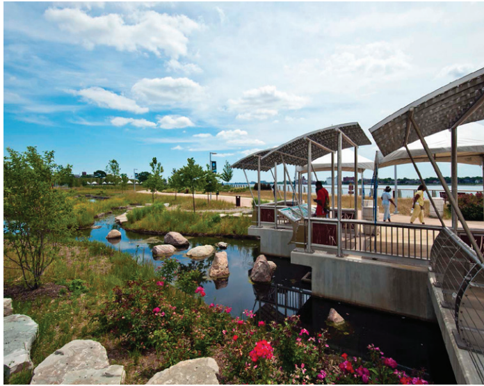
CONSTRUCTED WETLAND FILTERING 4.5 MILLION GALLONS OF STORMWATER RUNOFF
