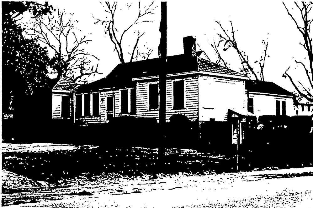
N.B. Young Preschool building (view southeast) from Black Archives, Research Center and Museum
