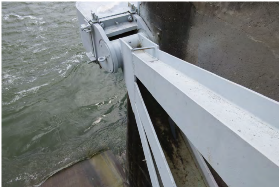
PHOTOGRAPH No.: 2 GATE: Gate 8 Photo Taken: 3/31/2020 File: MC-28.jpg
