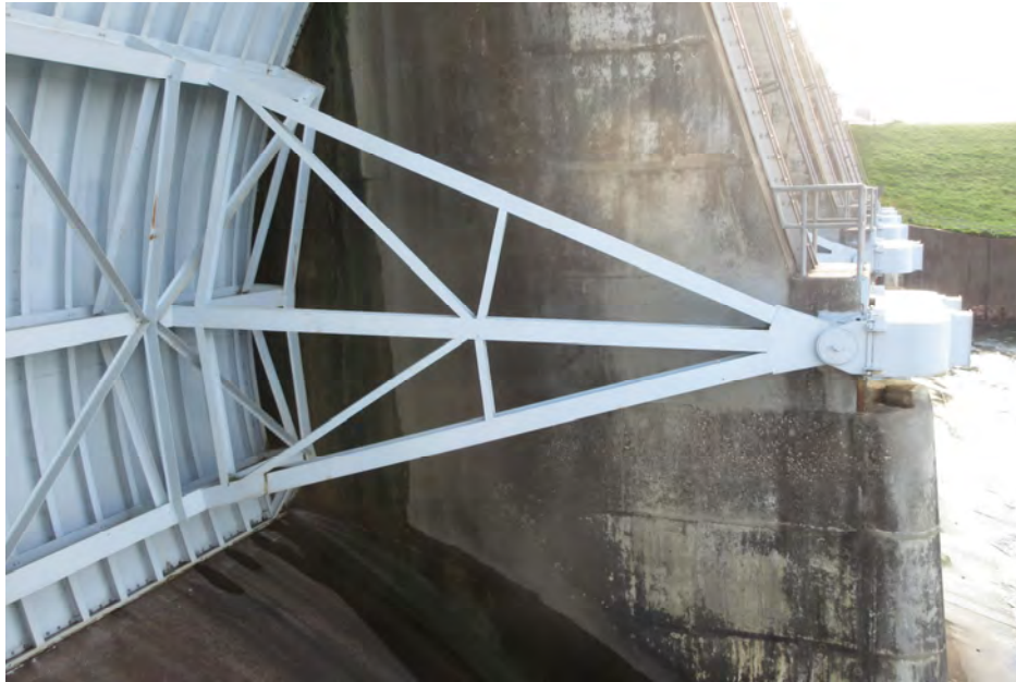
PHOTOGRAPH No.: 1 GATE: Gate 9 Photo Taken: 4/1/2020 File: MC-01.jpg
