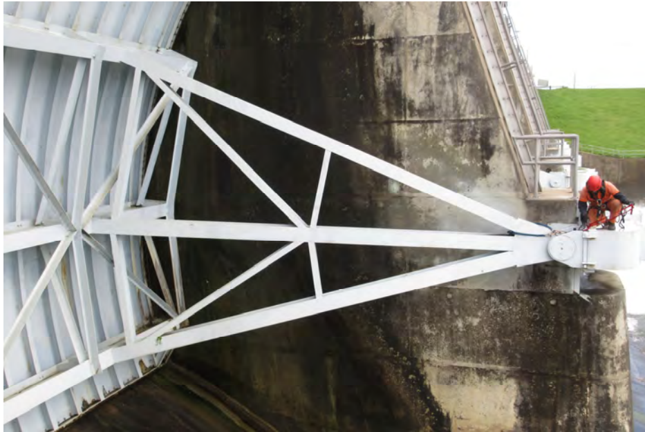
PHOTOGRAPH No.: 1 GATE: Gate 8 Photo Taken: 3/31/2020 File: MC-27.jpg
