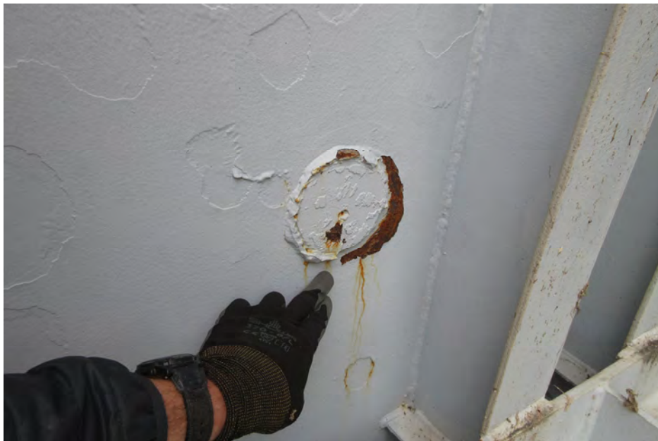
PHOTOGRAPH No.: 4 GATE: Gate 1 Photo Taken: 3/30/2020 File: MC-5.jpg
