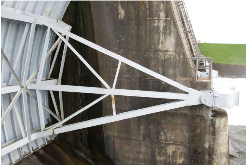
PHOTOGRAPH No.: 1 GATE: Gate 6 Photo Taken: 3/31/2020 File: MC-01.jpg
