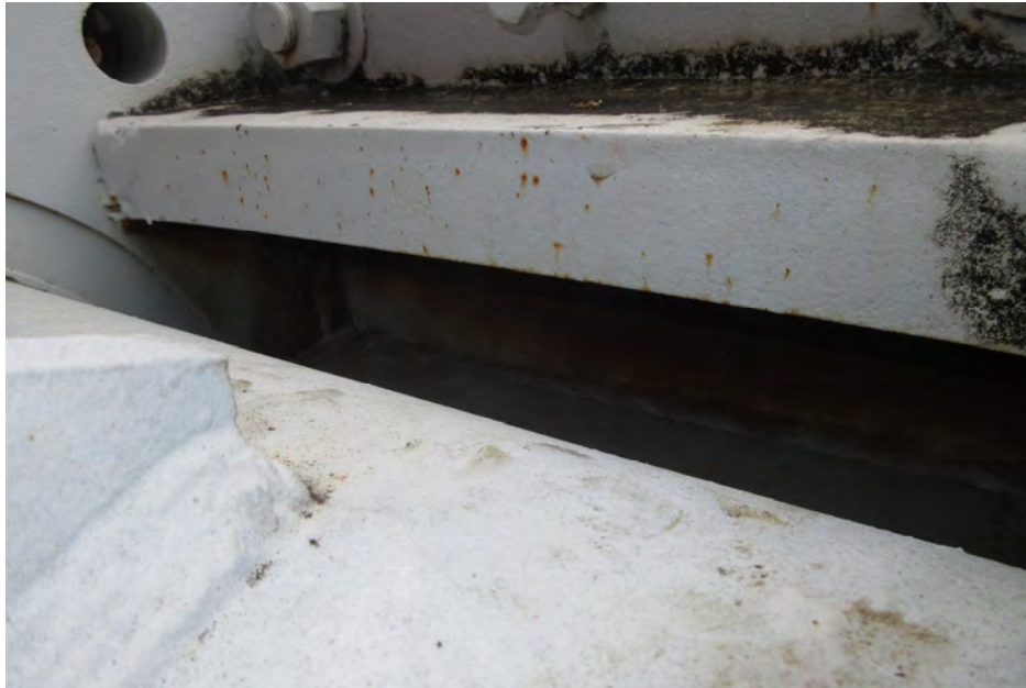
PHOTOGRAPH No.: 3 GATE: Gate 1 Photo Taken: 3/30/2020 File: MC-4.jpg
