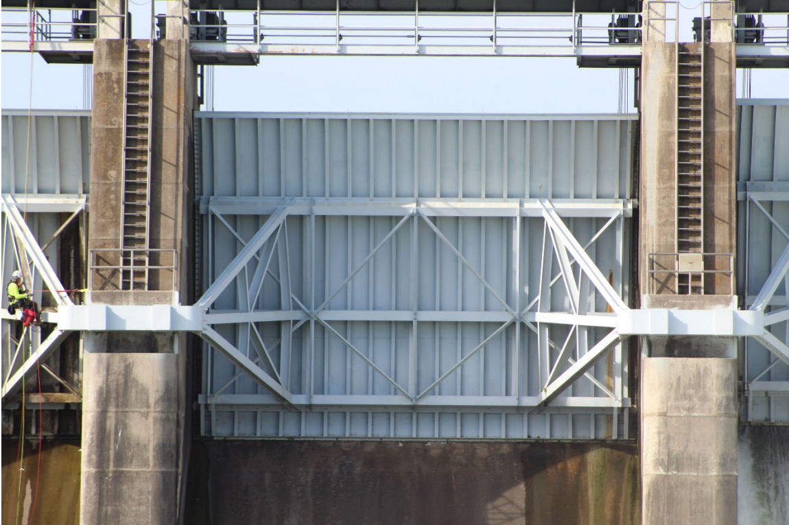
Photo 3-1: Downstream view of a Forney Dam Tainter gate.
