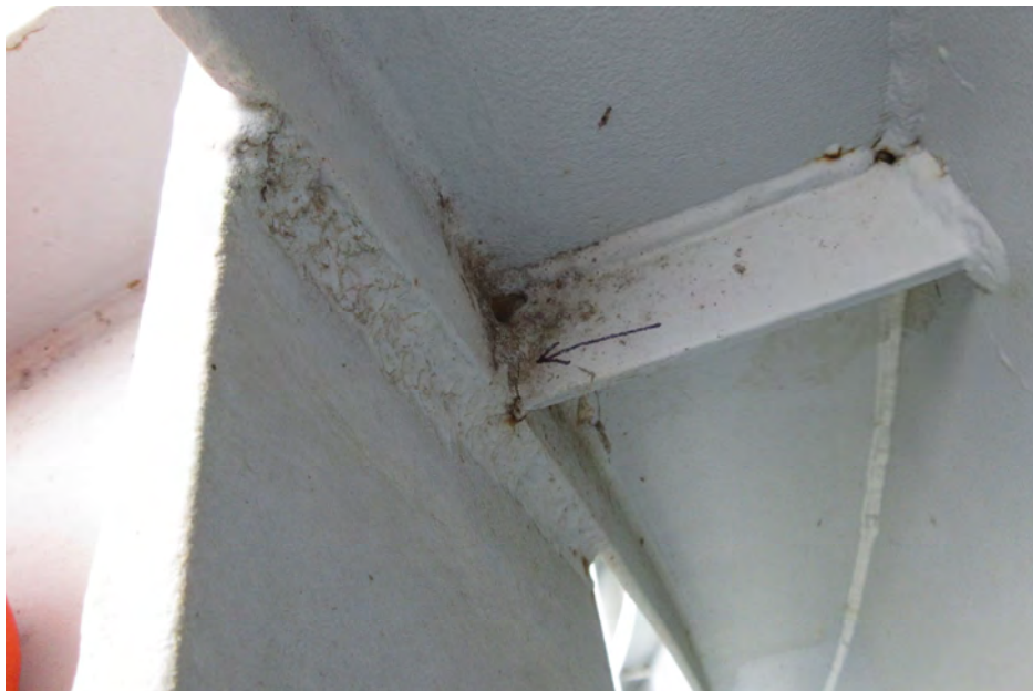
PHOTOGRAPH No.: 6 GATE: Gate 1 Photo Taken: 3/30/2020 File: MC-7.jpg
