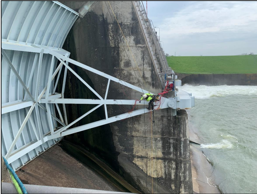
Figure 5 – BDI personnel installing instrumentation on the gate arm
