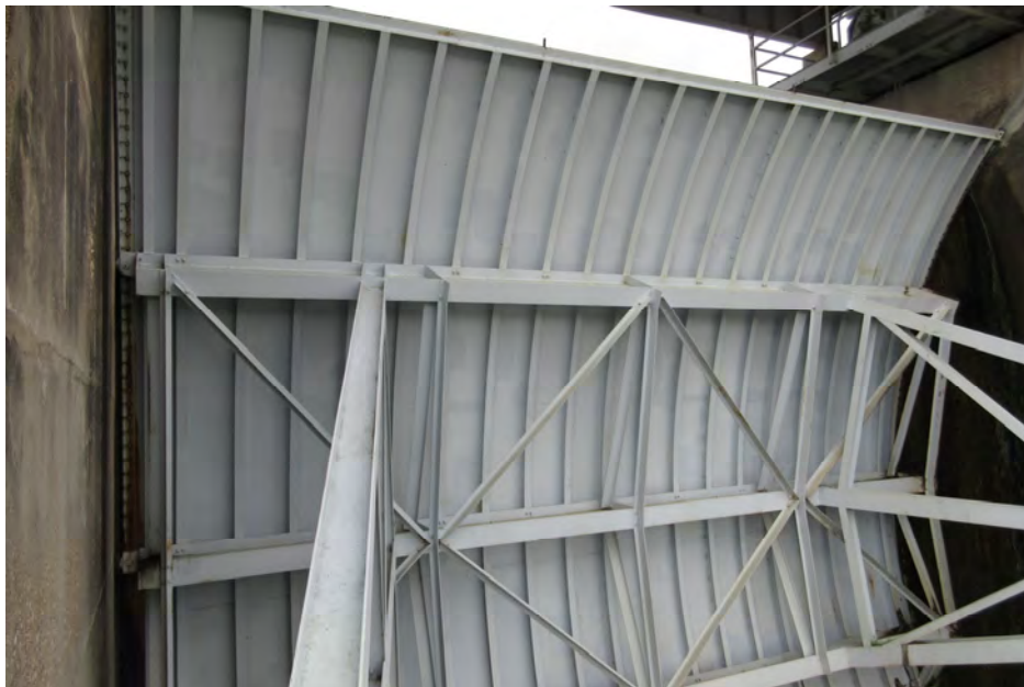
PHOTOGRAPH No.: 2 GATE: Gate 6 Photo Taken: 3/31/2020 File: MC-02.jpg
