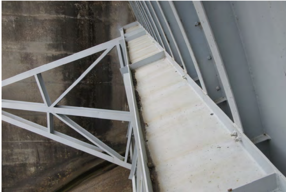
PHOTOGRAPH No.: 5 GATE: Gate 1 Photo Taken: 3/30/2020 File: MC-6.jpg
