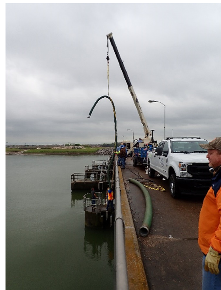
Photo 5-5: DWU Crews placing submersible pumps to de-water in front of Gate 6.
