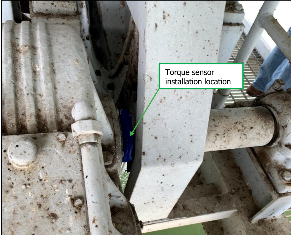
Figure 3 – Torque sensor installation on hoist pinion shaft (Typical)
