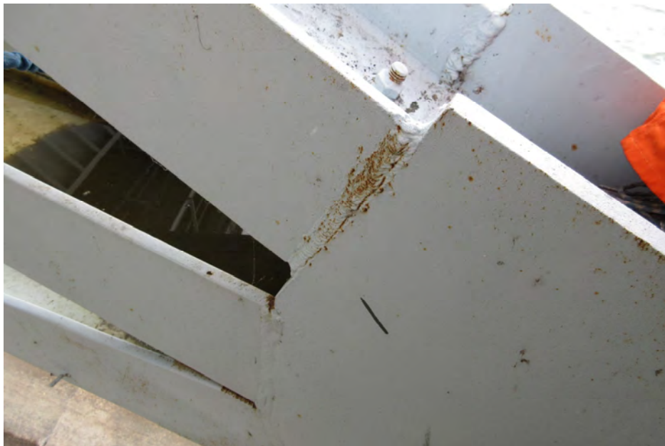
PHOTOGRAPH No.: 4 GATE: Gate 6 Photo Taken: 3/31/2020 File: MC-04.jpg
