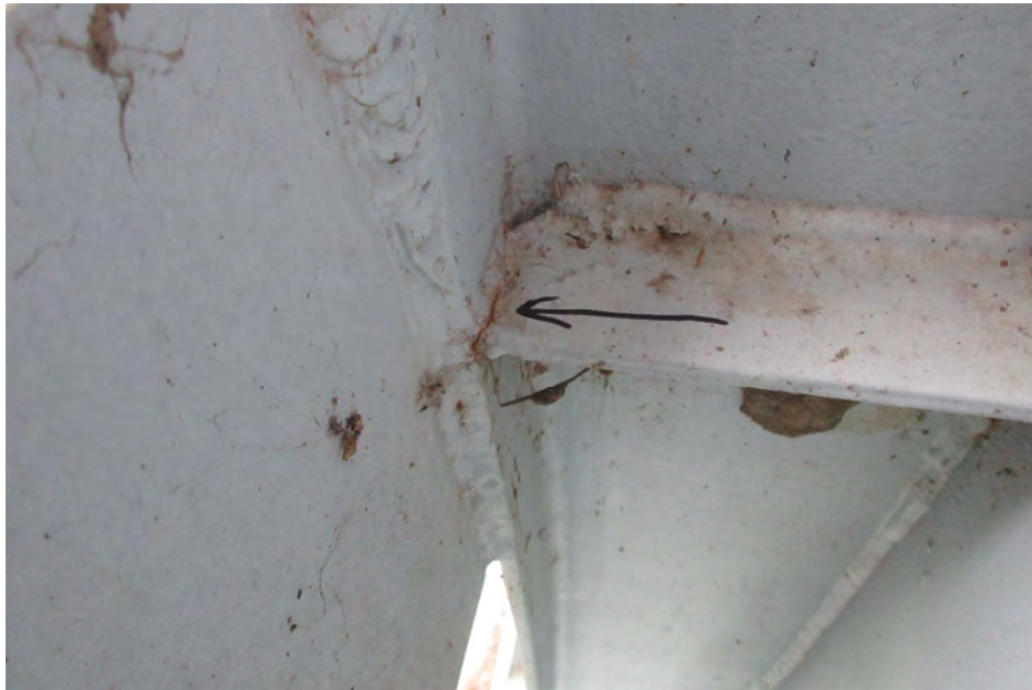
PHOTOGRAPH No.: 10 GATE: Gate 1 Photo Taken: 3/30/2020 File: MC-11.jpg
