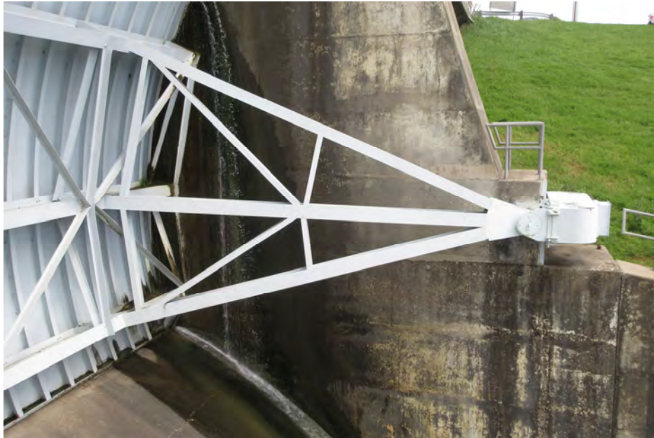
PHOTOGRAPH No.: 1 GATE: Gate 14 Photo Taken: 4/1/2020 File: MC-26.jpg
