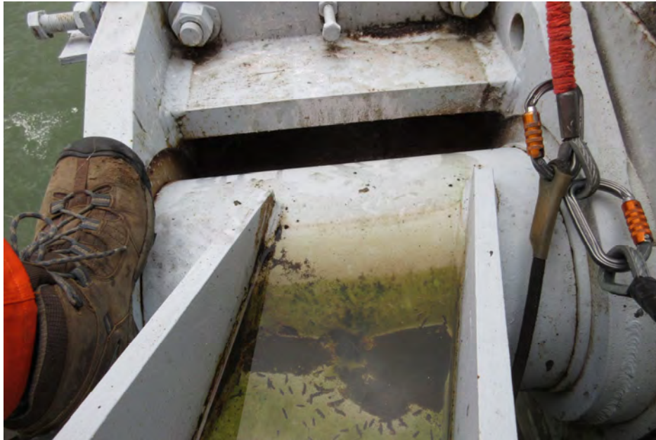
PHOTOGRAPH No.: 3 GATE: Gate 6 Photo Taken: 3/31/2020 File: MC-03.jpg
