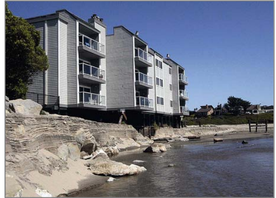
Figure 5-1: Erosion of low-lying area near Corcoran Lagoon Apartments. Source: Photo courtesy of the Santa Cruz Sentinel, 2011.
