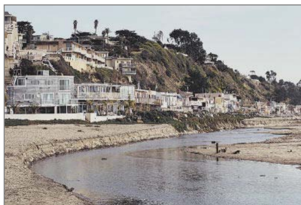
Figure 5-13: Rio Del Mar Beach Erosion Source: Santa Cruz Sentinel, January 2011.
