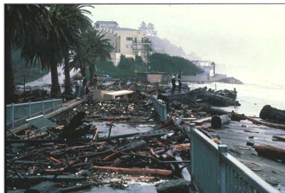
Figure 5-4: The Rio Del Mar Esplanade was damaged during the El Niño winter of 1983 by large waves arriving simultaneously with high tides and elevated sea levels. Source: Gary Griggs, University of California, Santa Cruz.
