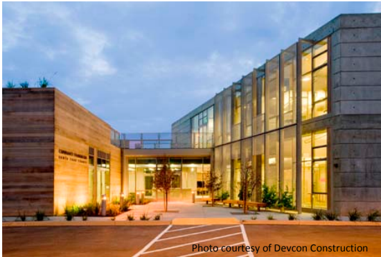
Photo courtesy of Devcon Construction
