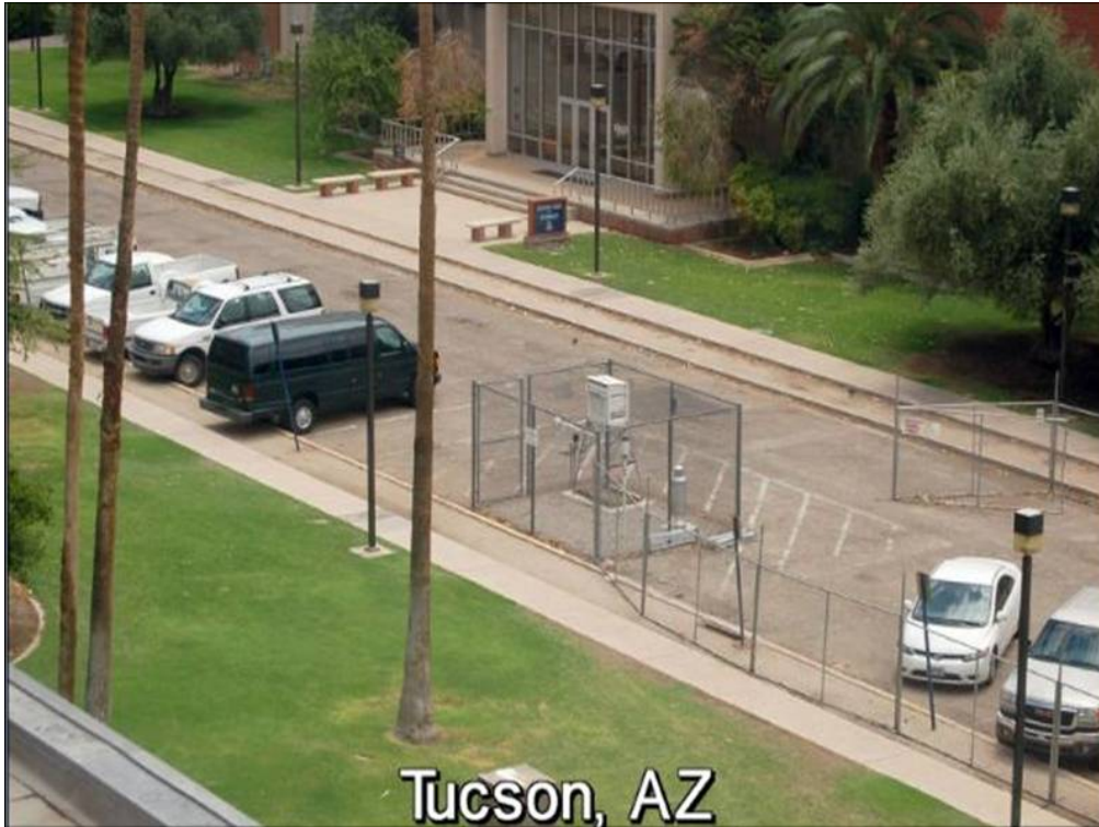
Tucson , Arizona in a parking lot on pavement.
