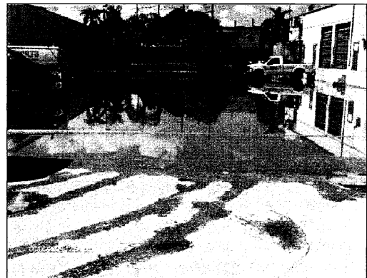
Nova solved localized flooding- NW 75 th Street- Medley
