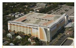
**PBC Parking Garage at Convention Center** Weitz pre-awarded the concrete shell package for the 9-story Palm Beach County Convention Center Garage to a shell subcontractor. By designing to the sub's concrete form system, Weitz saved more than \$1 million.
