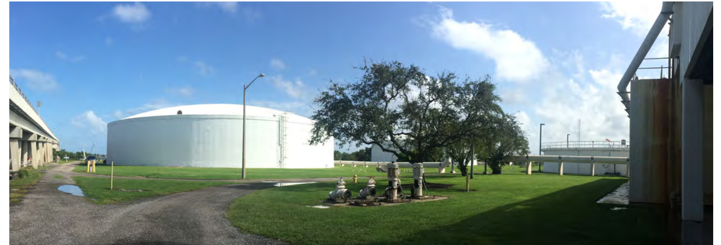
Water Treatment Tanks
