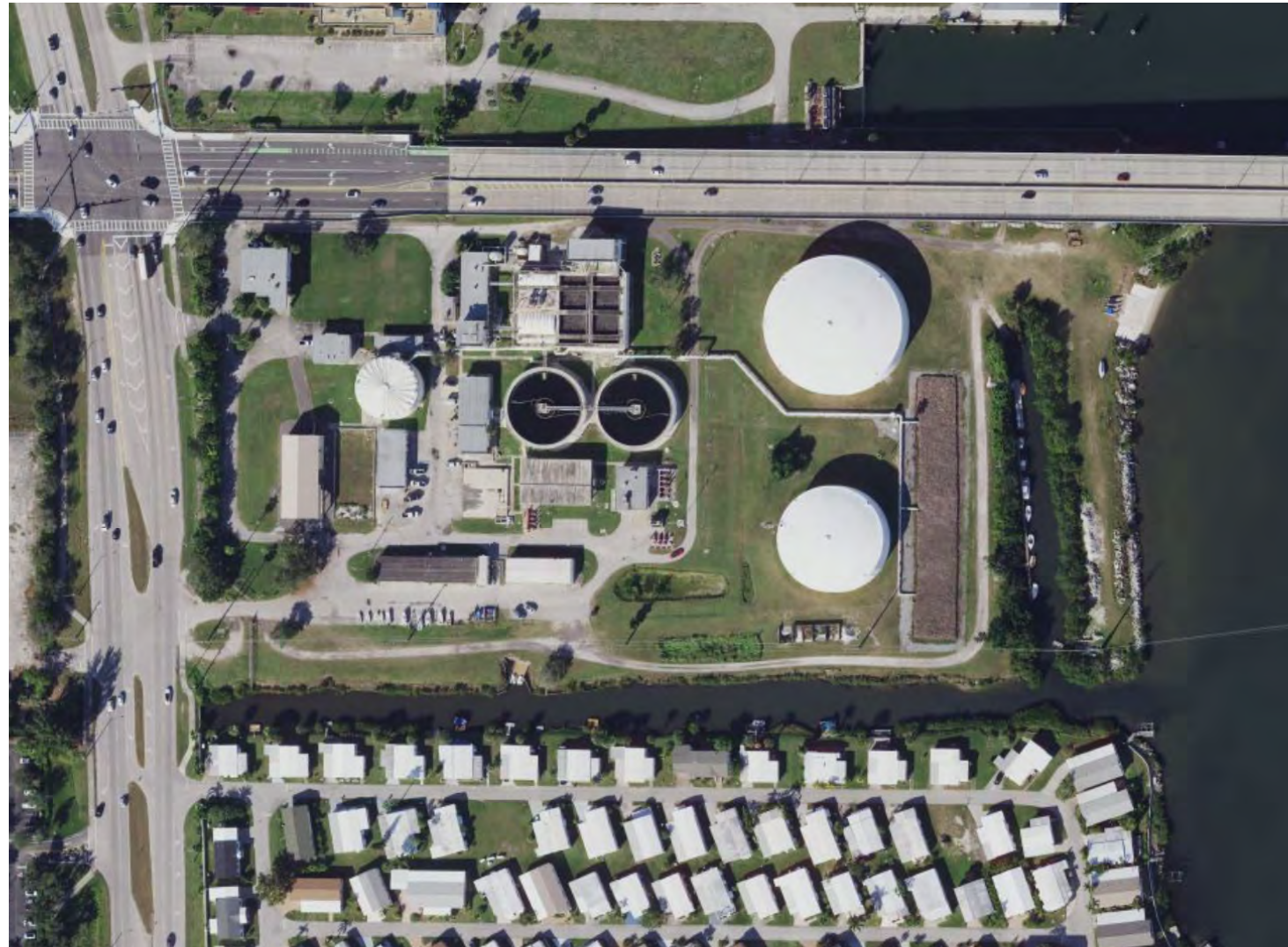
Water Treatment Plant Aerial
