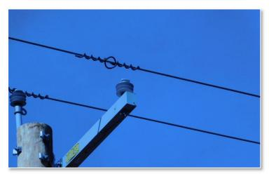
Below are conductors the Monitor team identified with splices tied in within 2' of an insulator.
