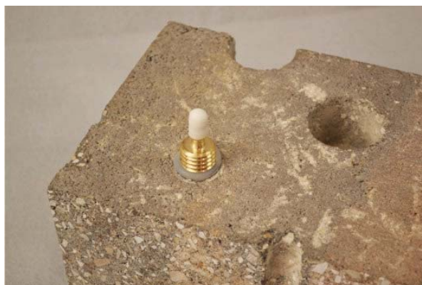
Figure 4. Installed Vapor Pin™.
