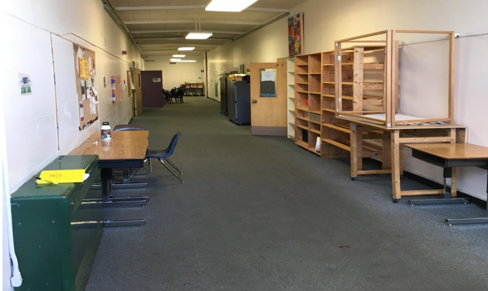
31. Annex Main Corridor – Discolored carpet.
