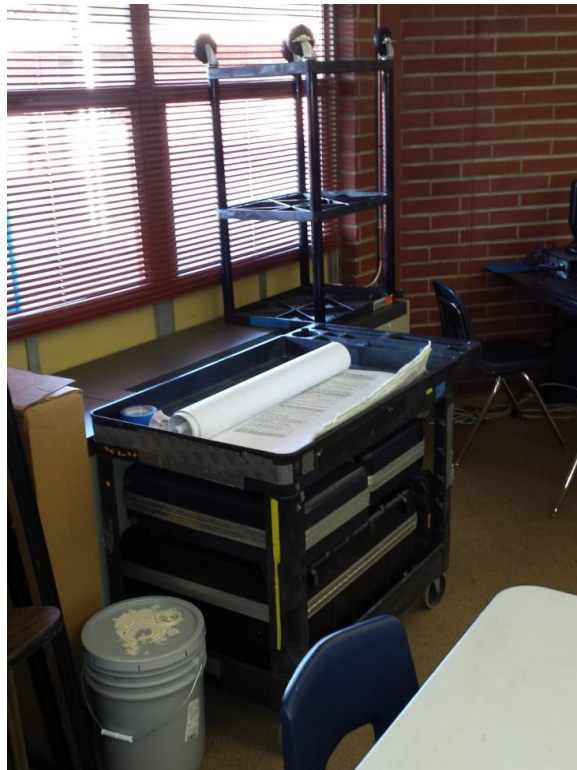
64. Classroom 1 – Items placed in front of and on top of the unit ventilator impeding air flow.
