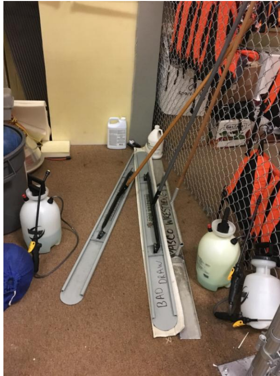
43. Small Gym Drama/Dance Storage – Leaking garden sprayers impacting carpet.
