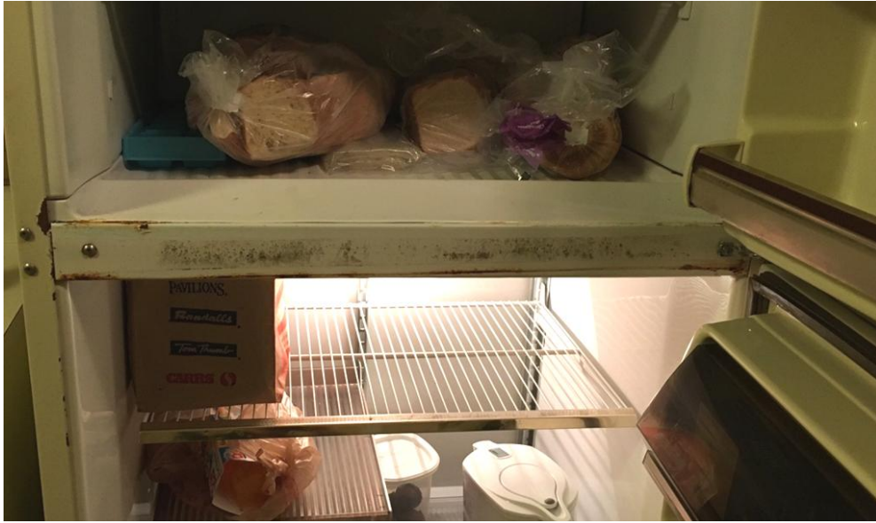
25. Annex 18-21 Transitions Kitchen – Moldy refrigerator door frame.
