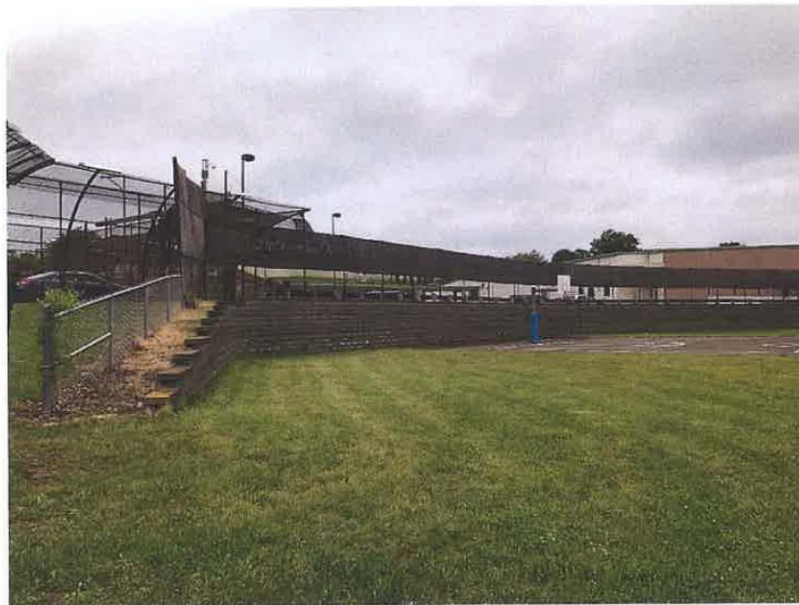
Photograph 2 –Retaining wall with Straight Fence. Secured Vehicular Entry in Background (Left)
