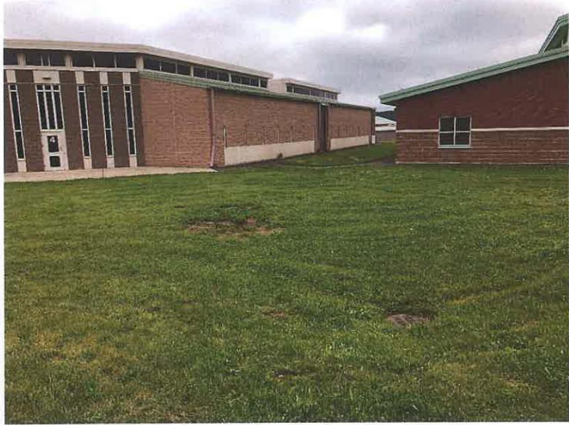
Photograph 4 – Building 4 (Left), Building 8 (Right)
