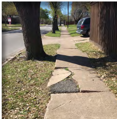
Figure 4. Examples of non-traversable sidewalks & ramps observed in the field
