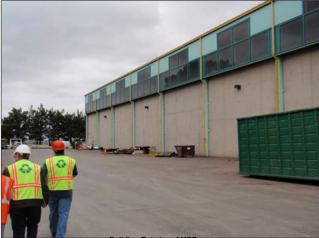
Building Exterior of MRF
