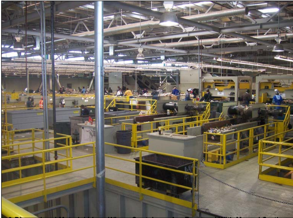
3-Dimensional Material Lines Where Containers Are Removed With Manual Sorting (Plastic & Glass), Cross Belt Magnets (Ferrous), and Eddy Current Separators (Aluminum Cans and Mixed Non-Ferrous)
