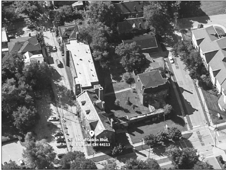
EXISTING SITE FROM ABOVE LOOKING SOUTH, CIRCA 2019
