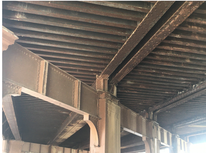
Steel underneath bridge
