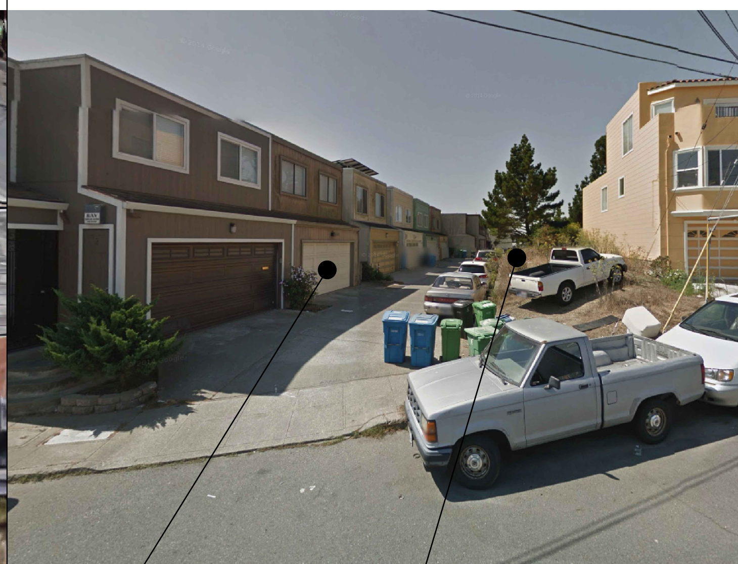
PROJECT LOCATION 8 MINERVA STREET REAR YARD VIEW
