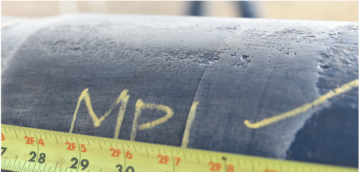
Figure 28: Shallow Metal Loss on Connection C014
