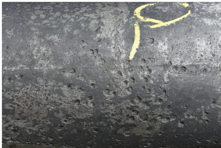
Figure 90: Type II Corrosion—Isolated Small Pits
