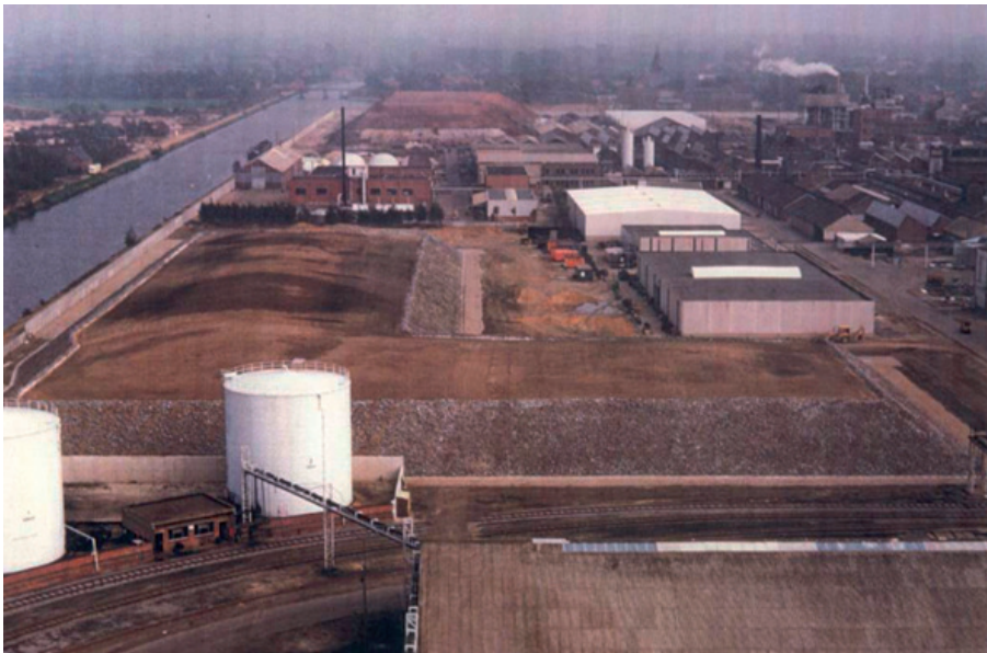
FIG. 7.8. View of the L-shaped UMTRAP facility at Union Minière, Olen.
