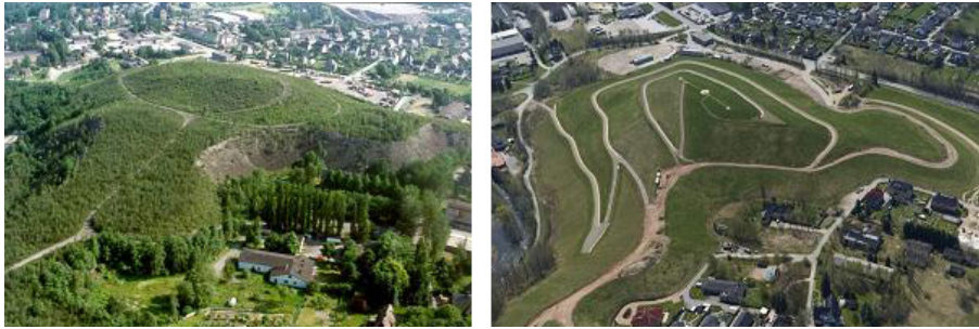
FIG. 7.18. Mine dump #66/207 at the Schlema site before and after cover placement.
