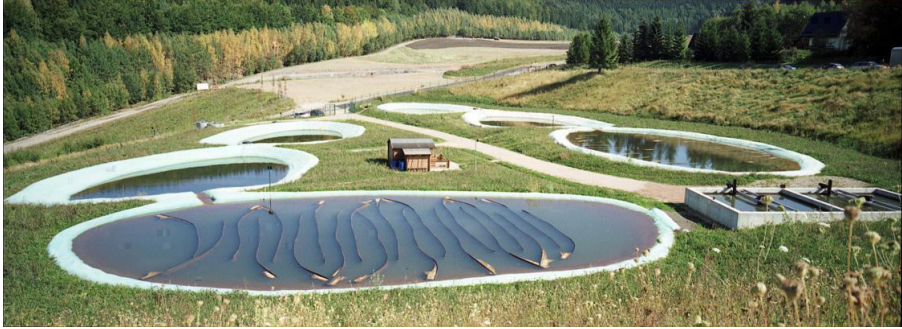
FIG. 7.22. Pilot scale unit for the passive treatment of flood waters from the Pöhla mine.
