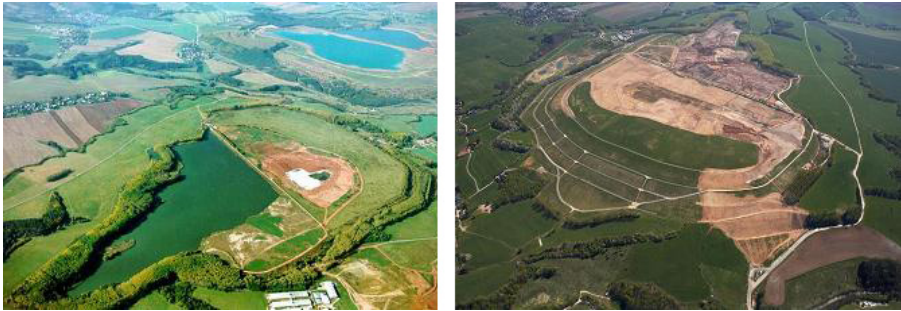
FIG. 7.20. Trünzig TMA before remediation was initiated and the present state of remedial progress at the site.
