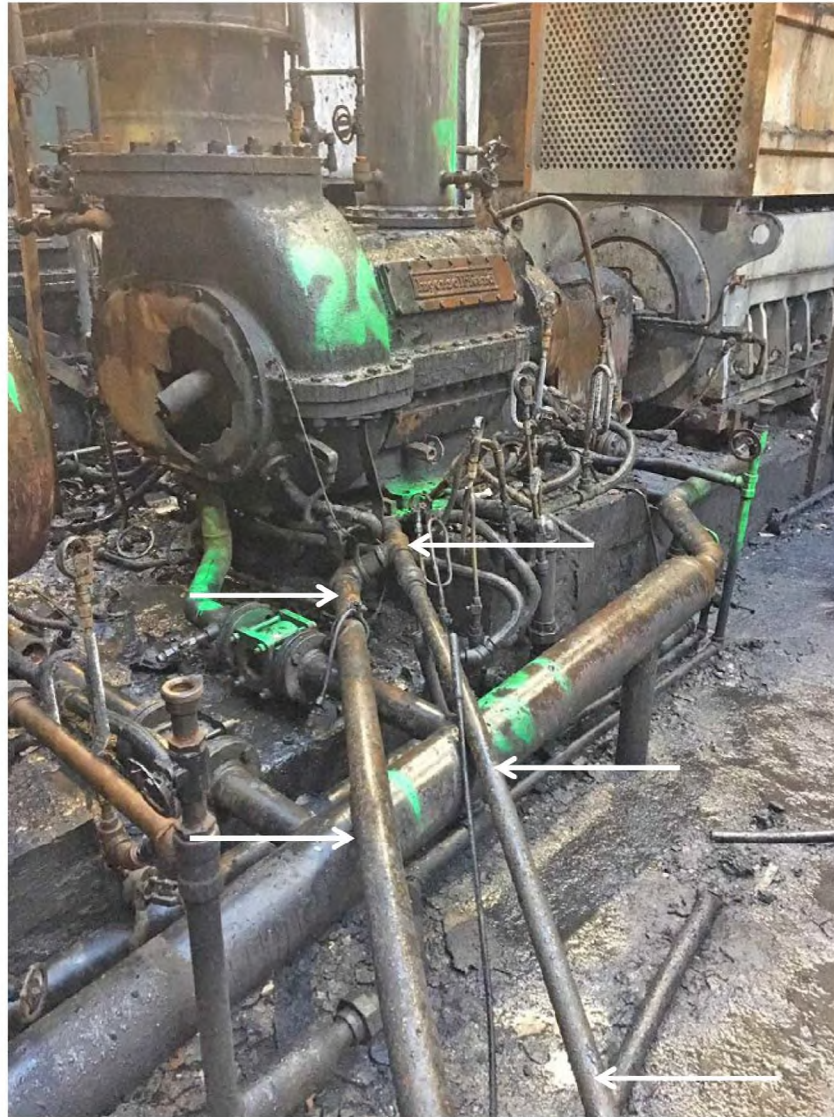
Photograph 4 - Pipe Section "C" – At C-521
