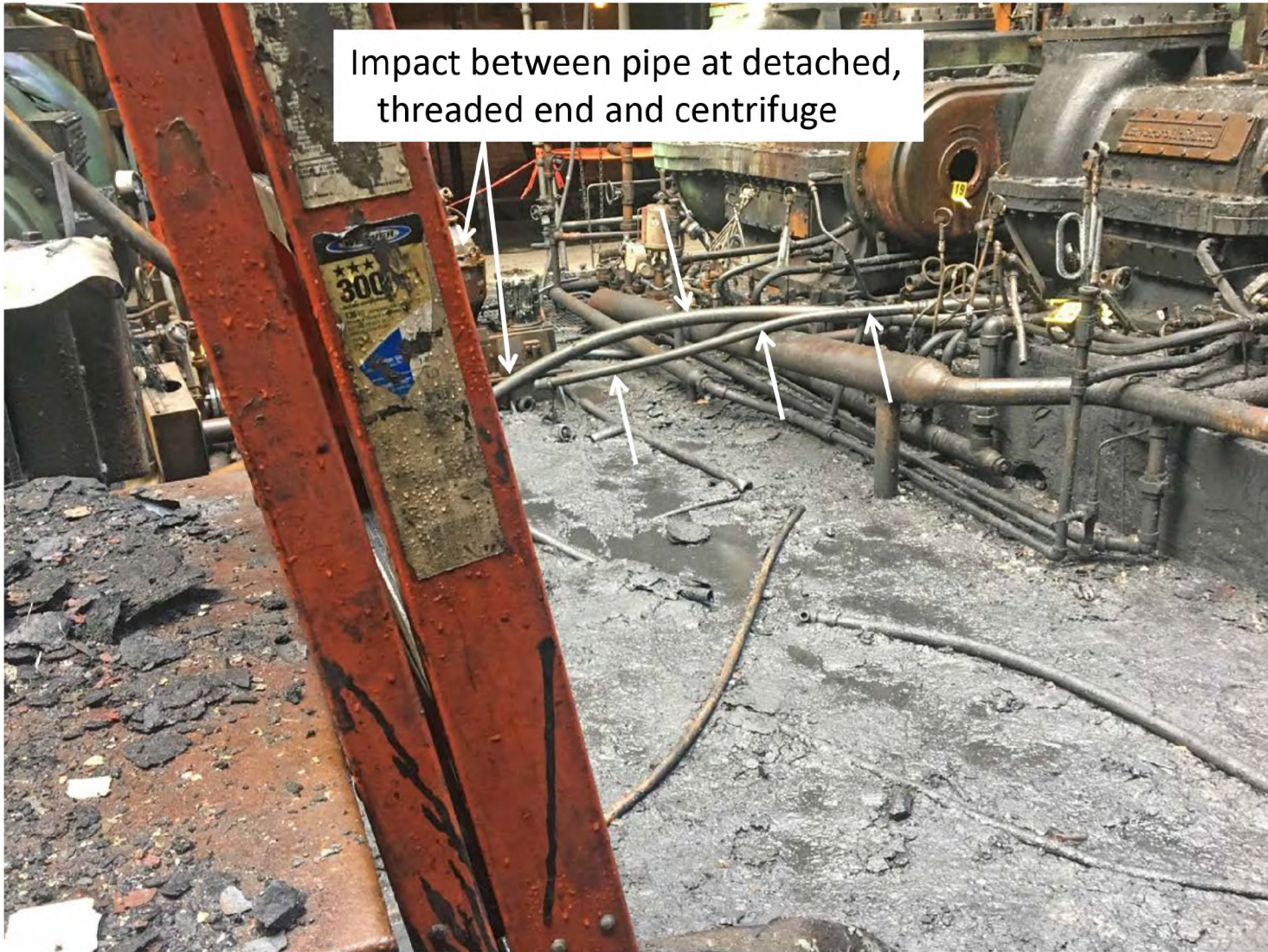
Photograph 5 - Pipe Section "C" – At C-521
