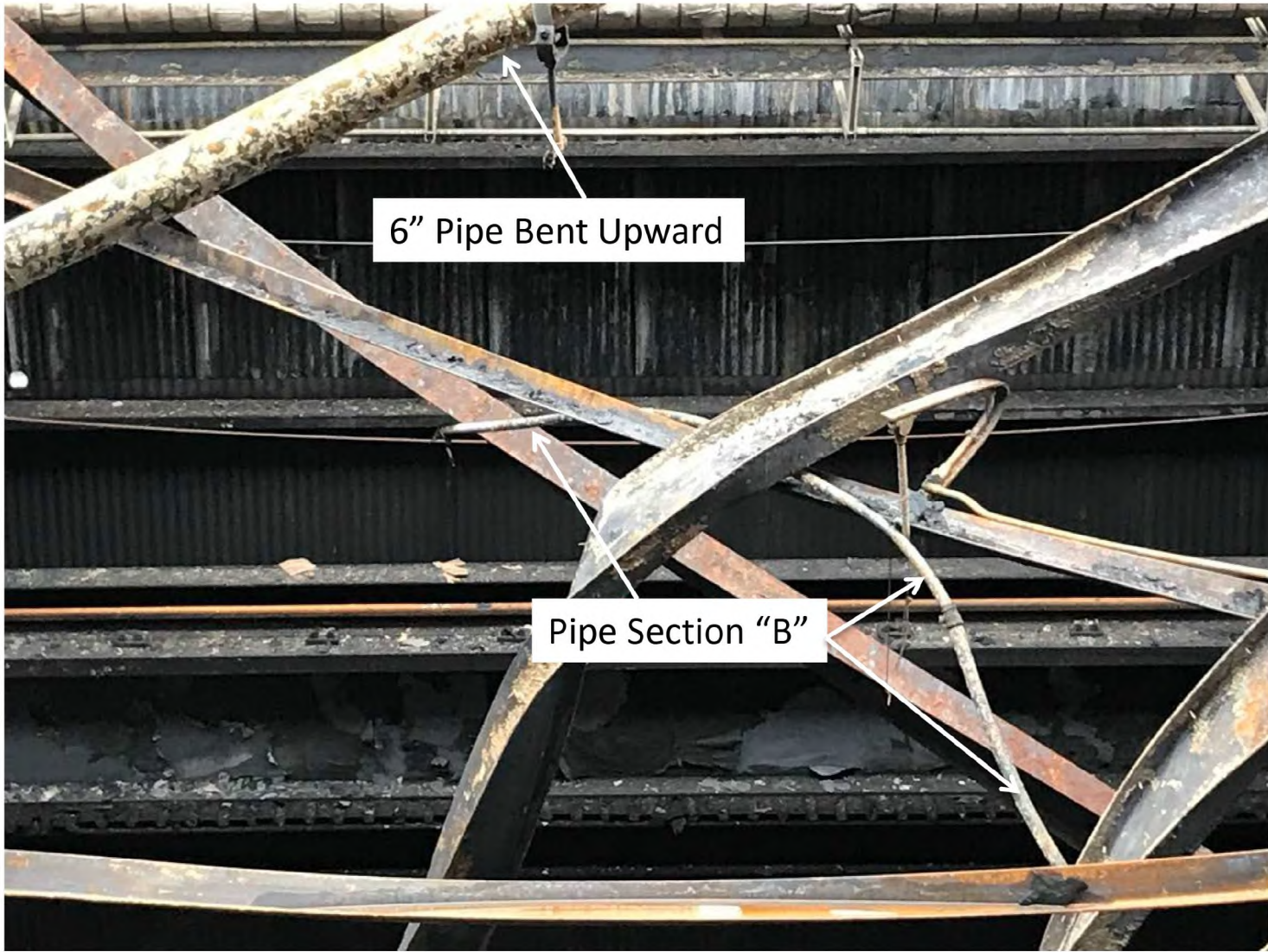
Photograph 3 – Pipe Section “B”
