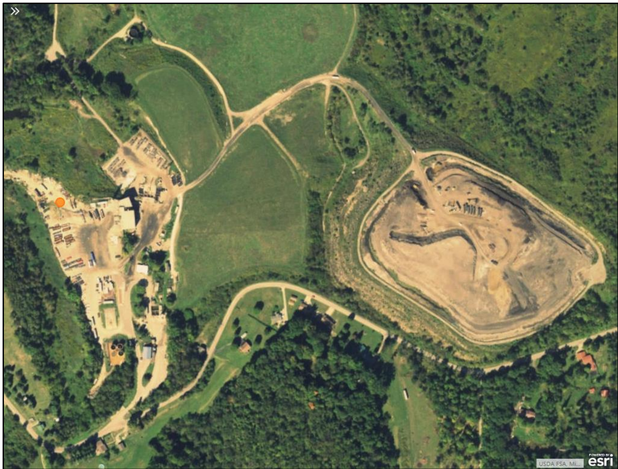
Figure 4-13. Aerial View of Max Environmental Technologies, Inc. Yukon Facility
