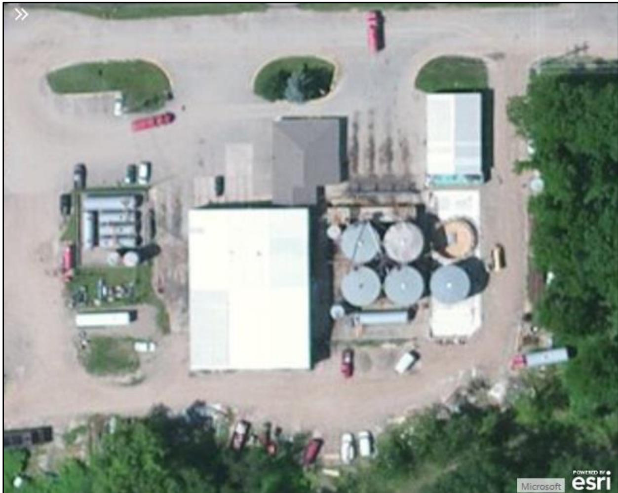
Figure 4-15. Aerial View of Waste Treatment Corporation Facility
