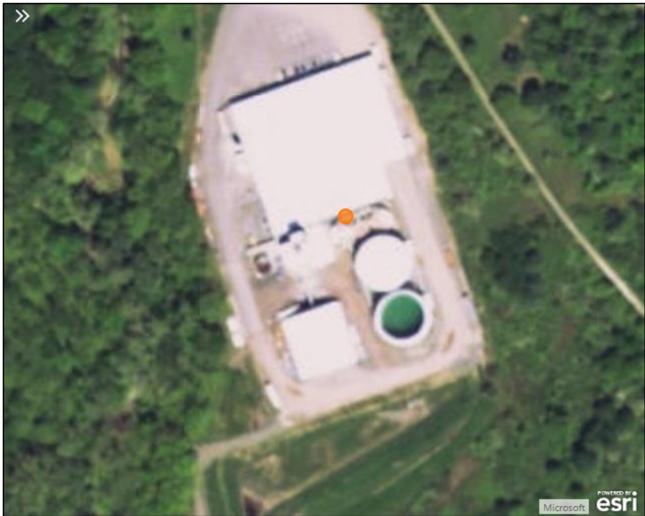
Figure 4-7. Aerial View of Eureka Standing Stone Facility
