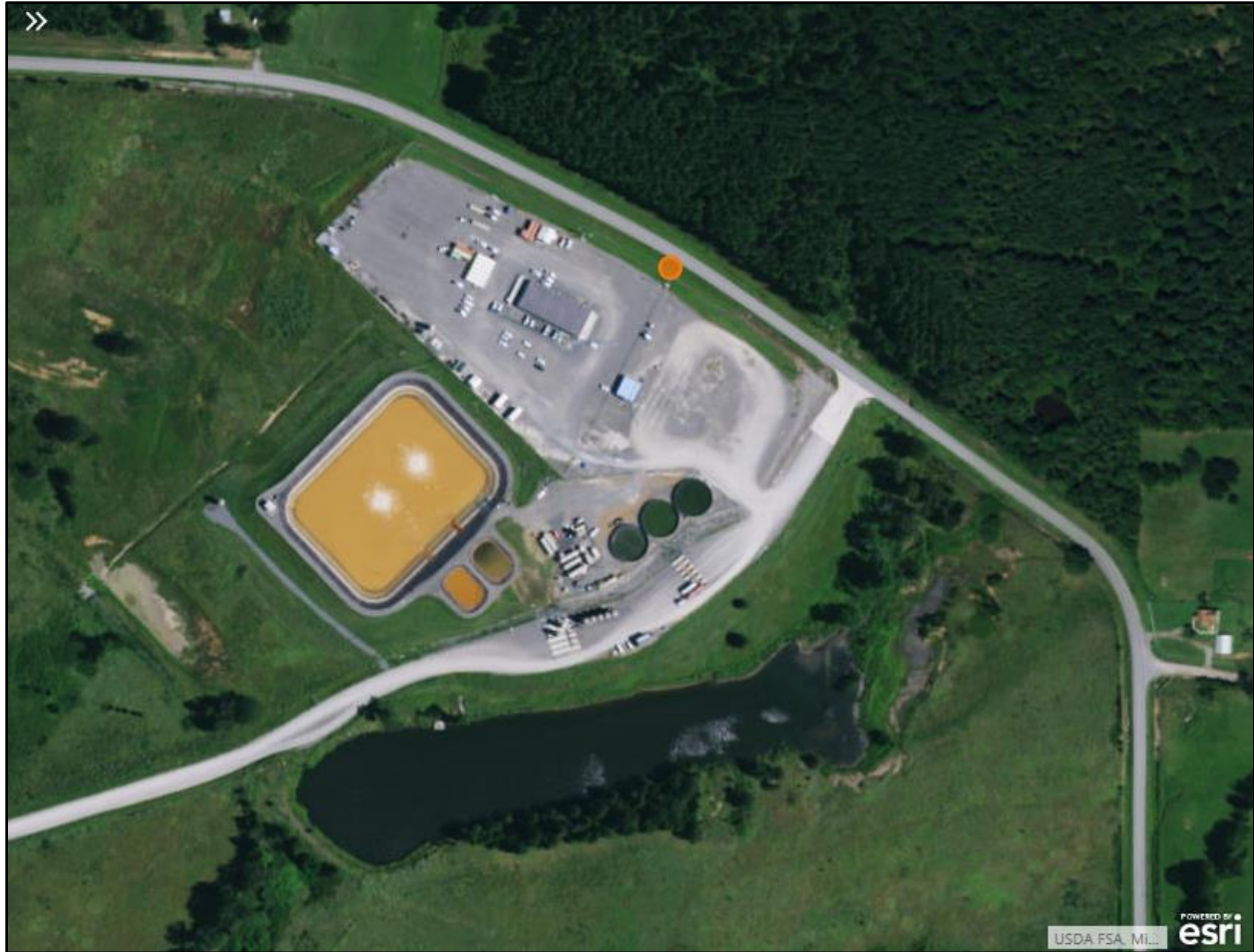
Figure 4-5. Aerial View of Judsonia Treatment Facility
