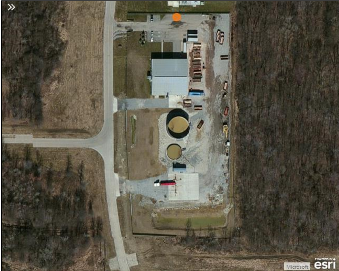
Figure 4-14. Aerial View of Patriot Water Treatment, LLC Facility
