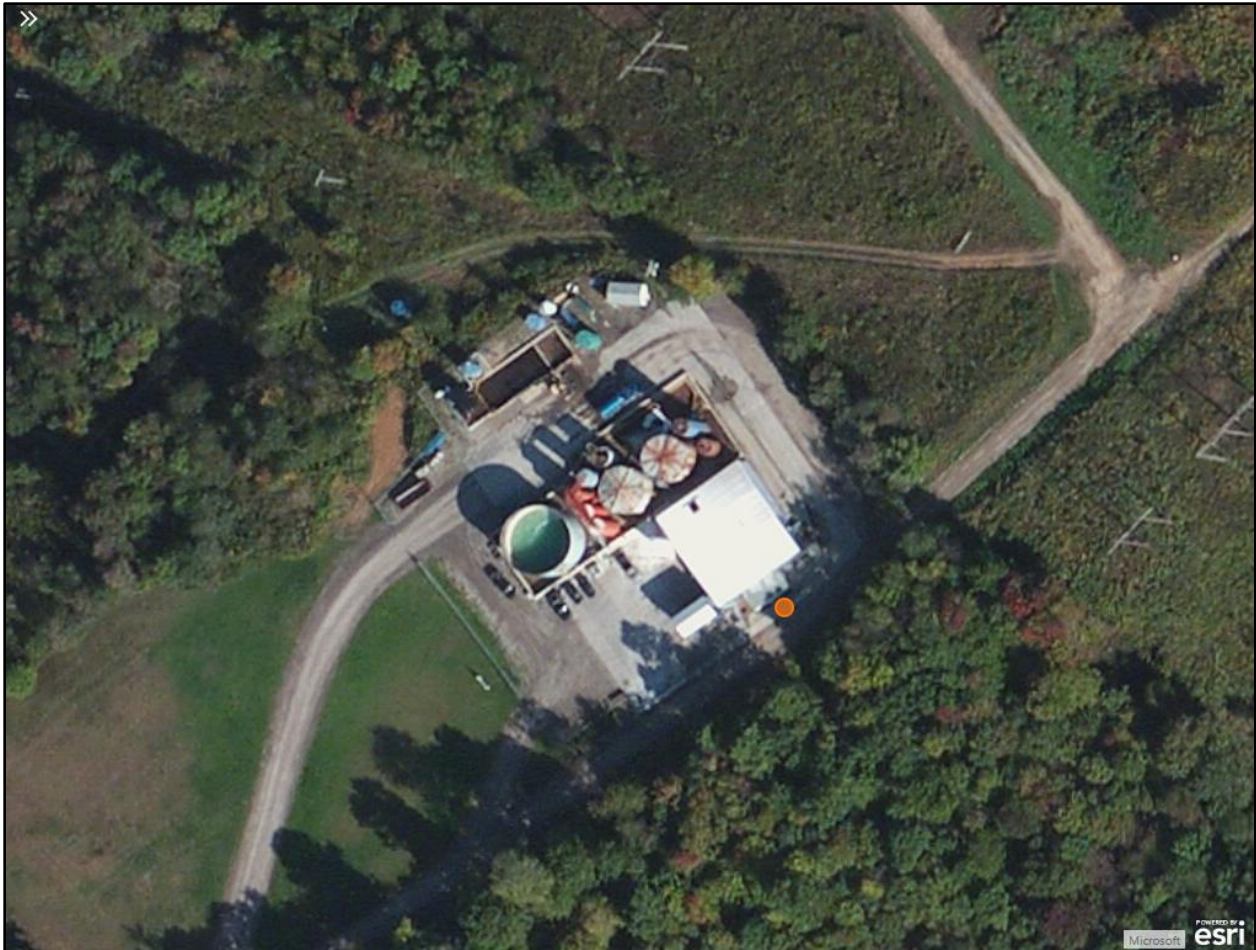
Figure 4-11. Aerial View of Fluid Recovery Services Josephine Facility
