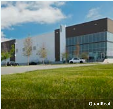
QuadReal's Nose Creek Business Park, Rocky View County, Alberta, features a sustainable and energy efficient design
