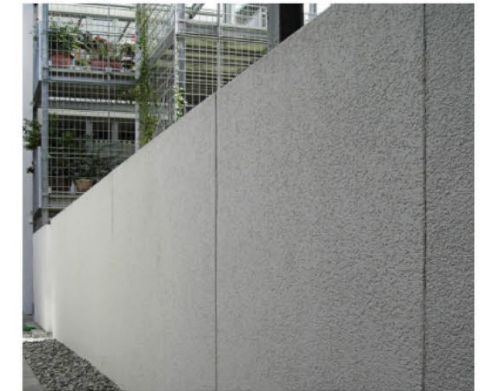
TAPERED ARCHITECTURAL FINISH CONCRETE WALL
