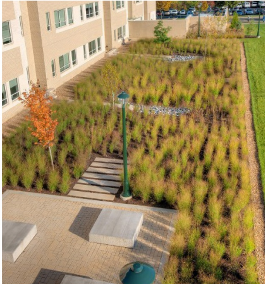
RAIN GARDEN MEADOW PLANTING, CONCRETE WEIRS AND DRY BED STONES AND BOULDERS
