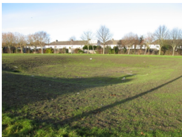
Fig 4.1: Swales Constructed at Glendhu Park, Cabra
