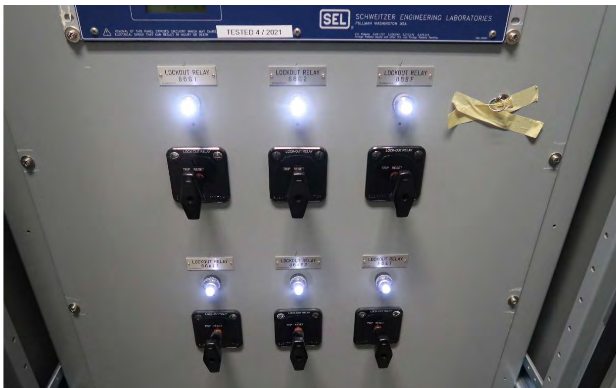
Photograph 12, STG 86 Series Lockouts Trip/Reset levers
