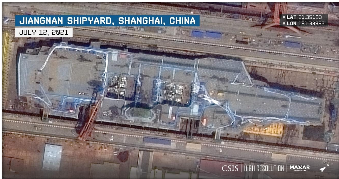
Figure 11. Type 003 Aircraft Carrier Under Construction
