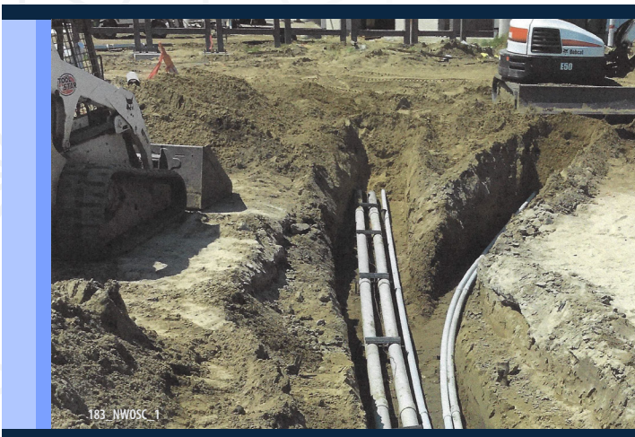
Malone Electrical in the field installing fiber and telephone infrastructure conduits at the airport in New Orleans.
