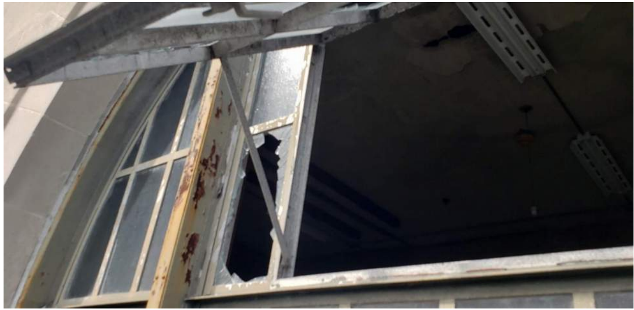
Photo 41: Window A. Operable Unit.
