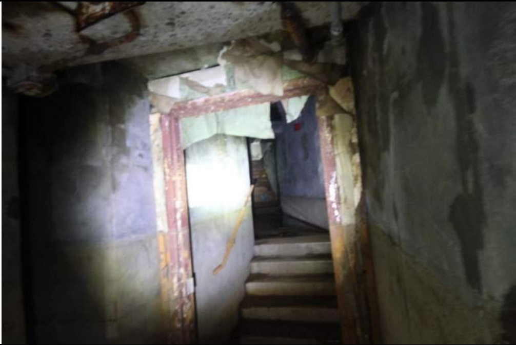
Photo 1: Basement Passageway to First Floor Stairs
