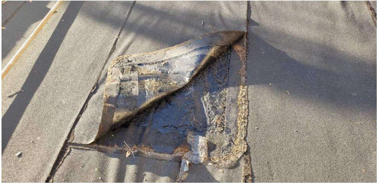
Photo 97: Field Membrane of Roof D
