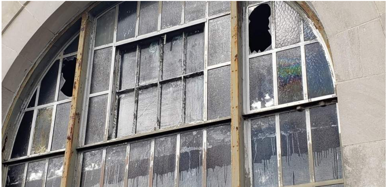
Photo 40: Window A. Operable Unit.
