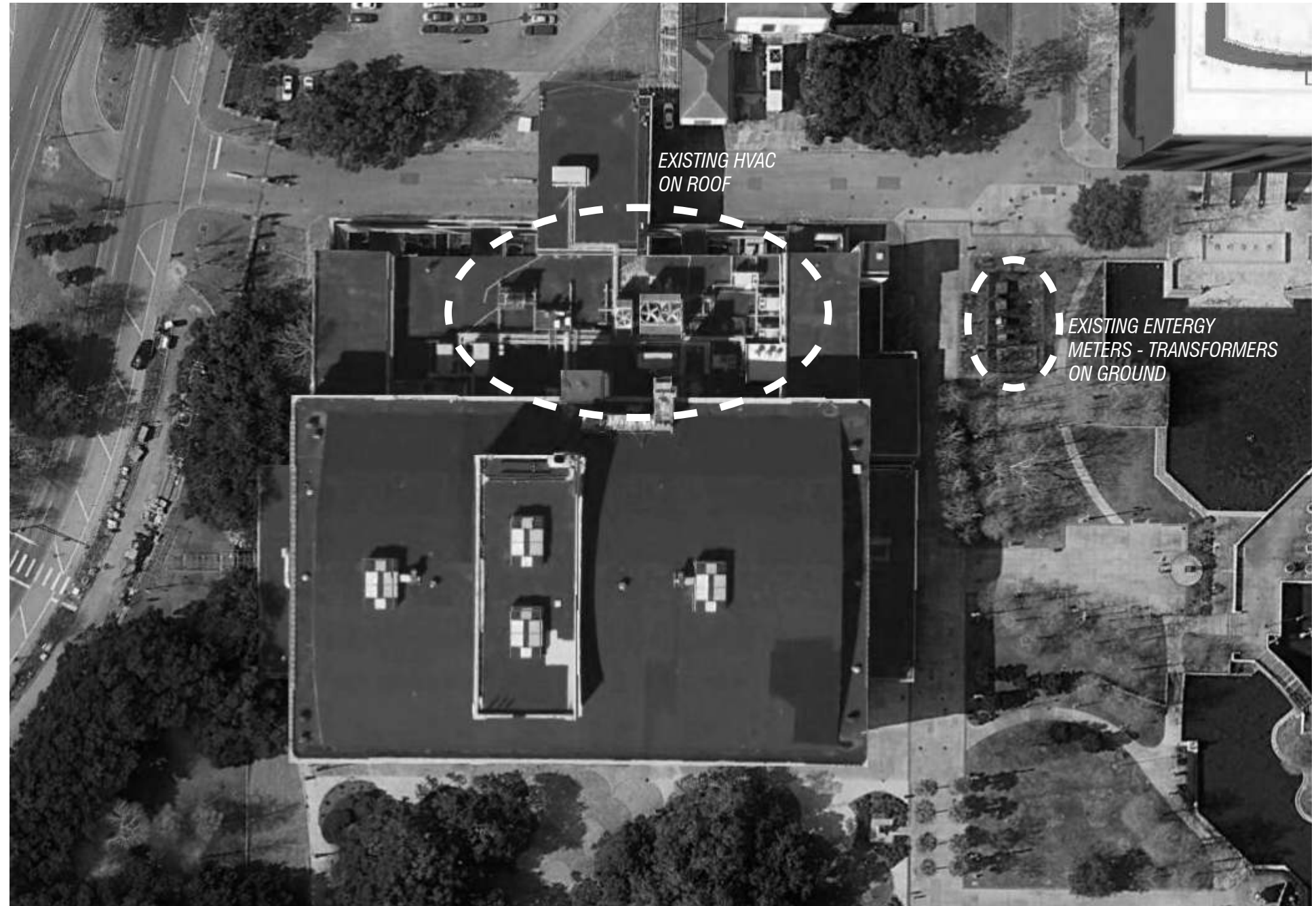
AERIAL VIEW OF MUNICIPAL AUDITORIUM SHOWING LOCATION OF EXISTING MEP SYSTEMS.
