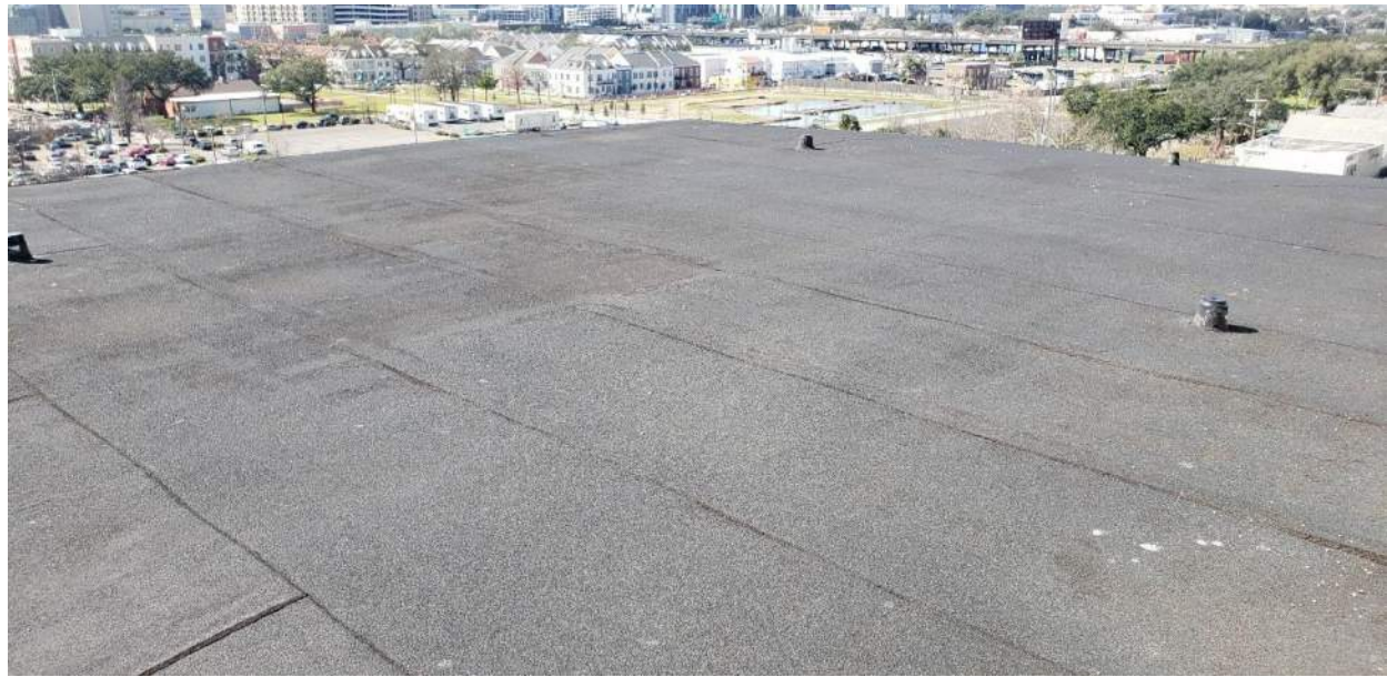
Photo 57: Field of Barrel Vault Roof
