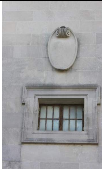
Photo 28: Type J: Masonry Opng. Steel Casement Opng. Out"
