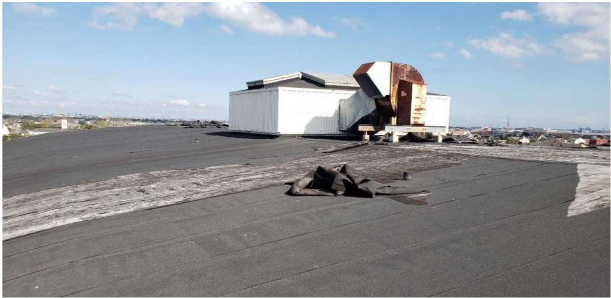
Photo 51: Skylight Well atop Barrel Vault Roof
