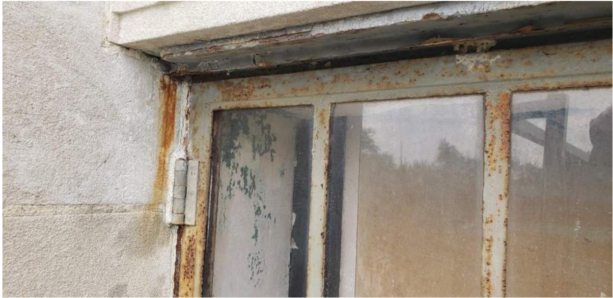
Photo 45: Window C Top Corner @ Area A @ N. Rampart Elevation
