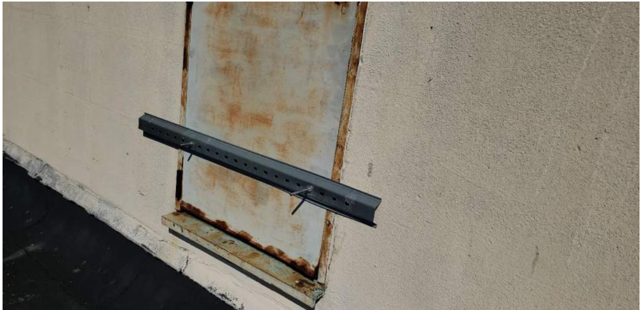
Photo 90: Roof Access Door
