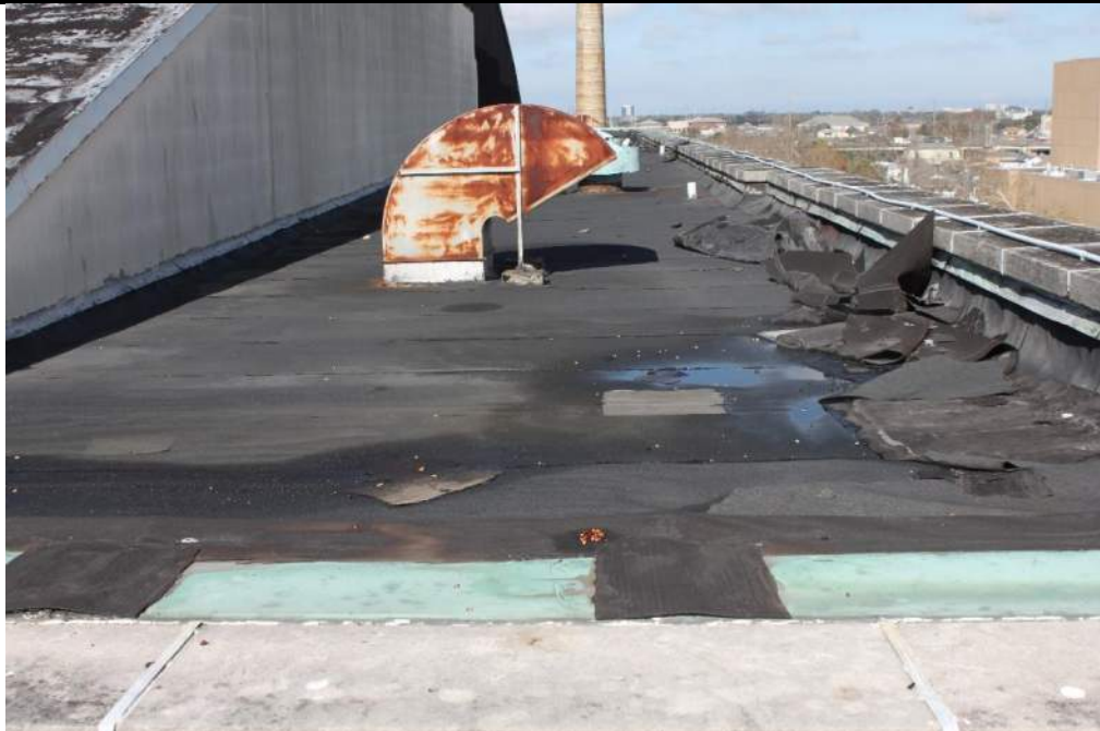
Photo 9: Flat Portion at St. Ann Street side between Gable and Coping
