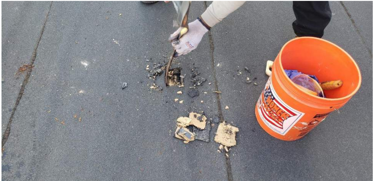
Photo 80: Roof E Area Drain
