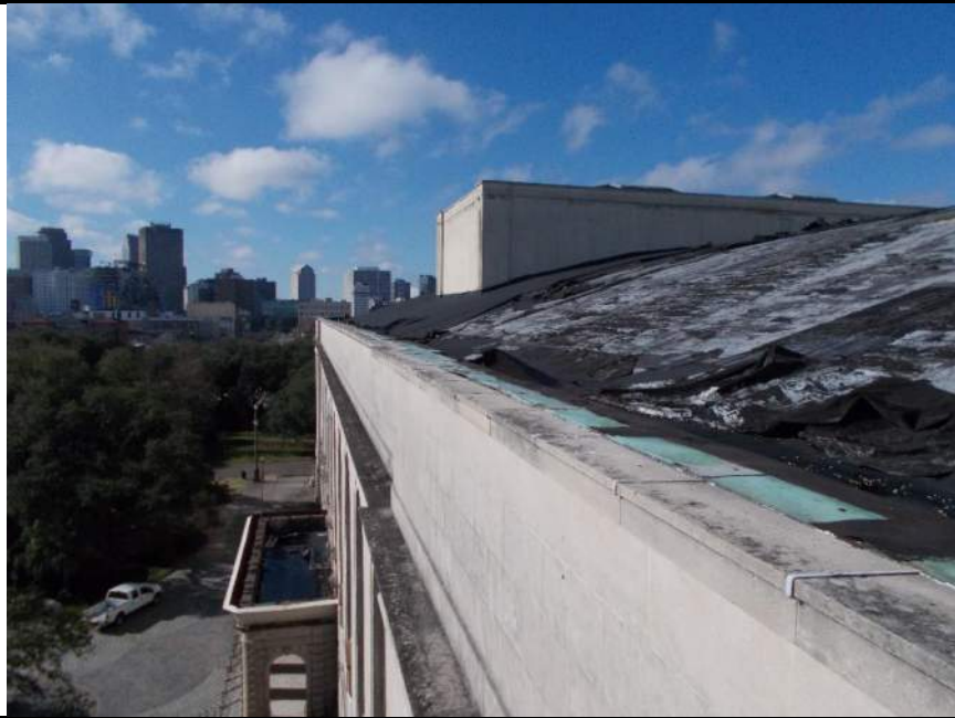
Photo 63: Parapet Along N. Rampart
