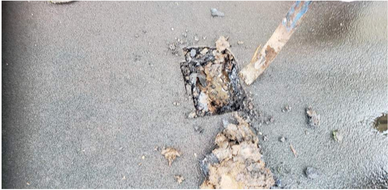
Photo 81: Roof E - Core #1
