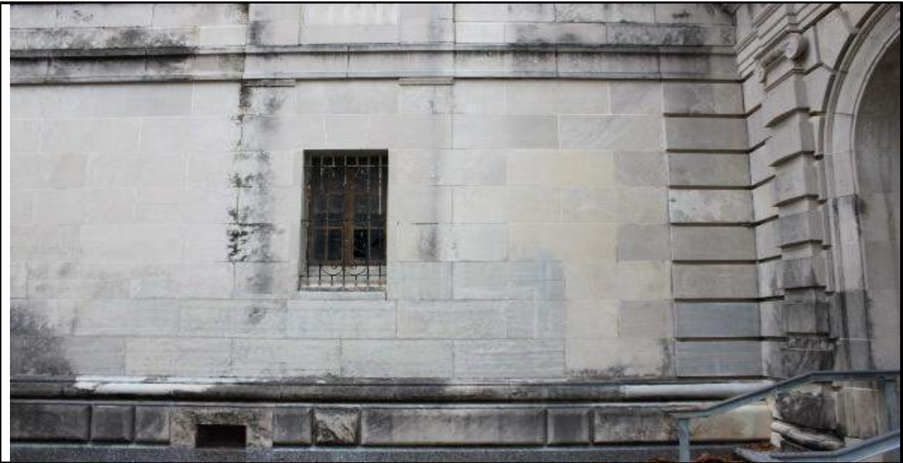
Photo 27: TYPE G "Masonry Opng. Steel Casement Opng. Out"
