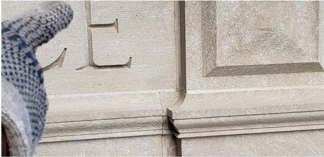
Photo 85: Cracking Limestone
