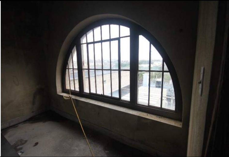
Photo 31: Type B: “Circular Headed Masonry Openings – Steel Sash and Frame”
