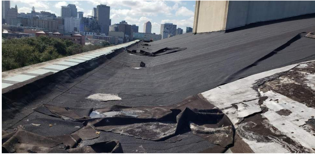
Photo 49: Roof Valley Along N. Rampart
