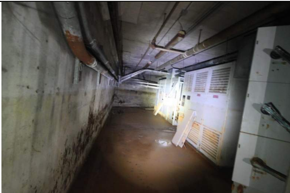
Photo 6: Rear Wall of Basement towards St. Ann Street
