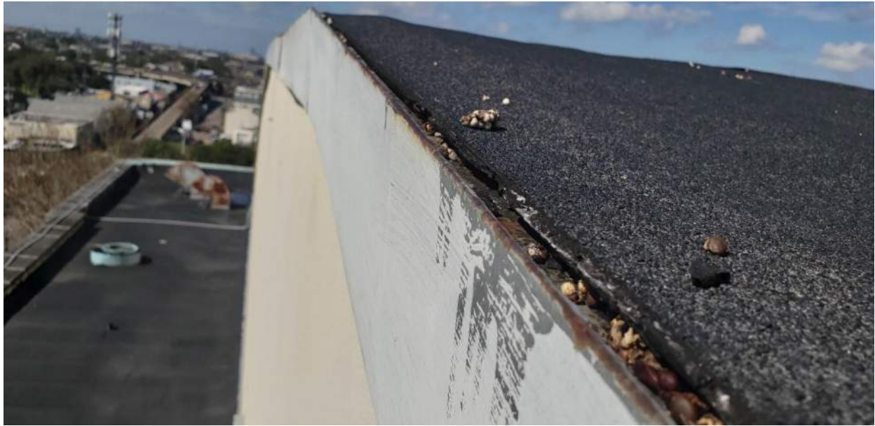
Photo 55: Edge Condition along Barrel Vault Rake
