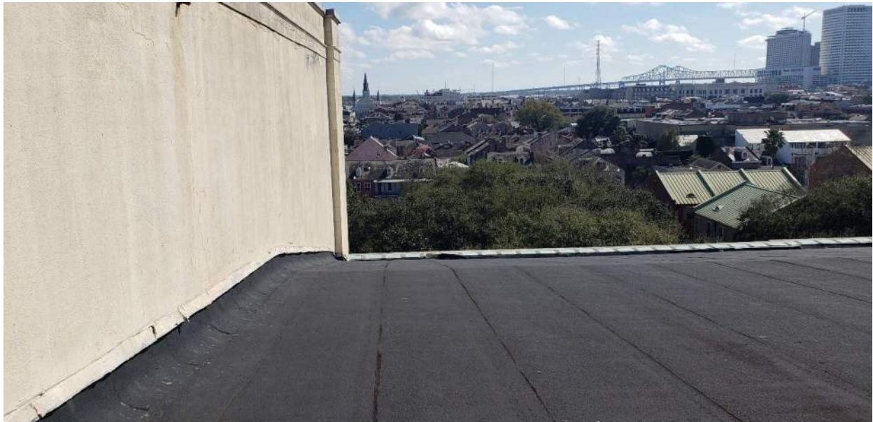
Photo 56: Barrel Vault @ Stage House (Area B)
