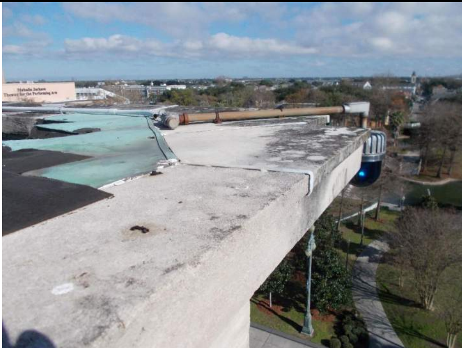
Photo 64: Parapet @ N. Rampart and St. Ann
