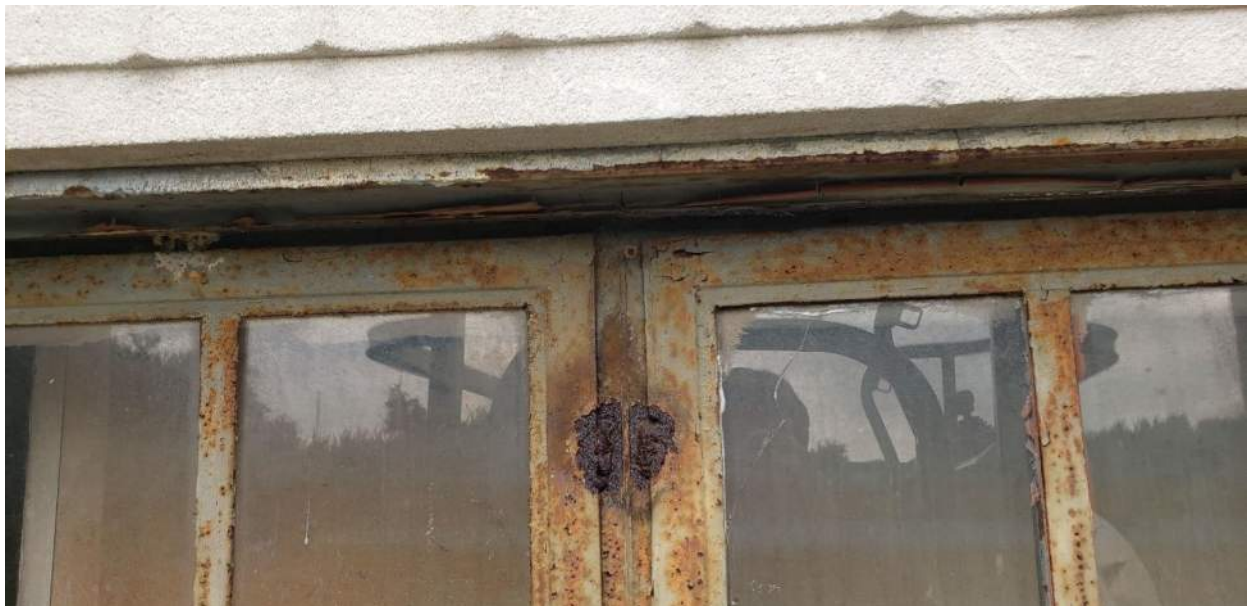
Photo 44: Window C Head @ Area A @ N. Rampart Elevation
