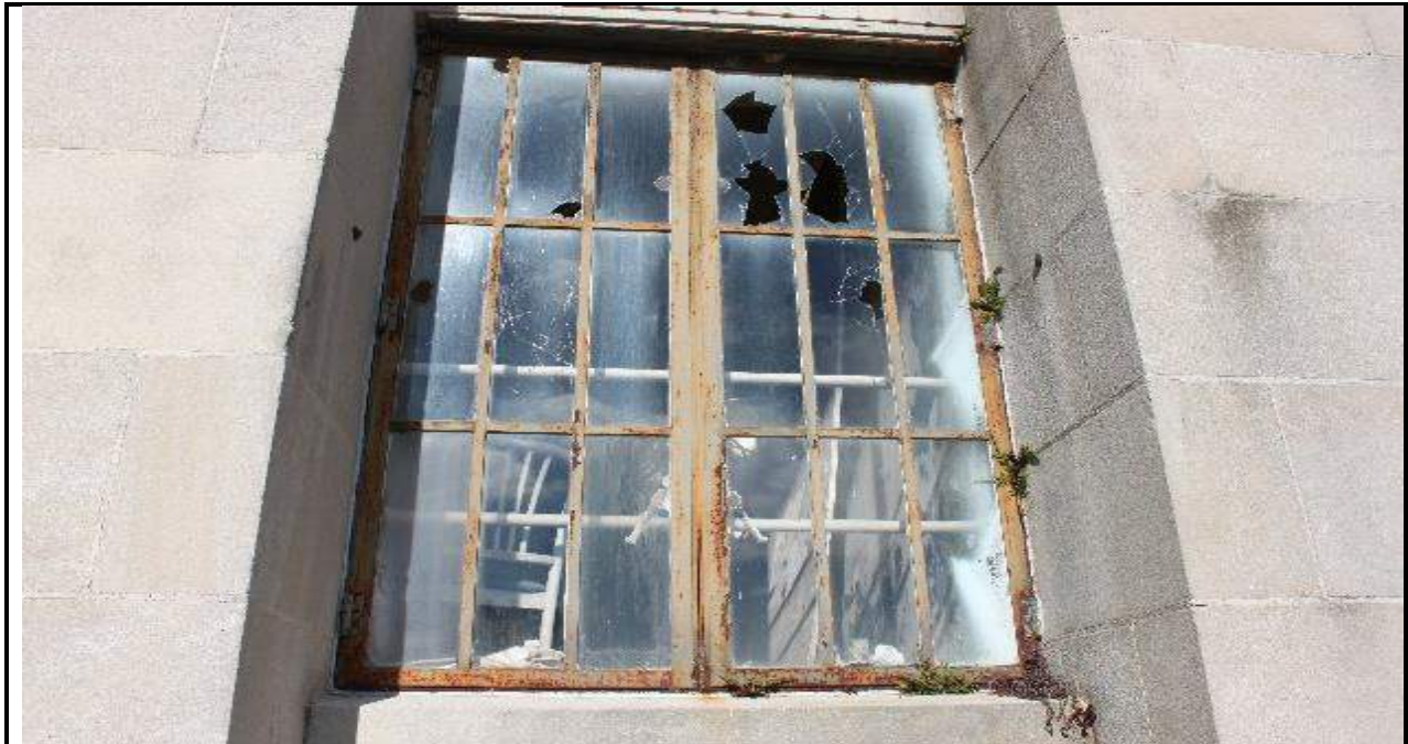
Photo 25: Type C: "Masonry Opng. Steel Casement Opng. Out"
