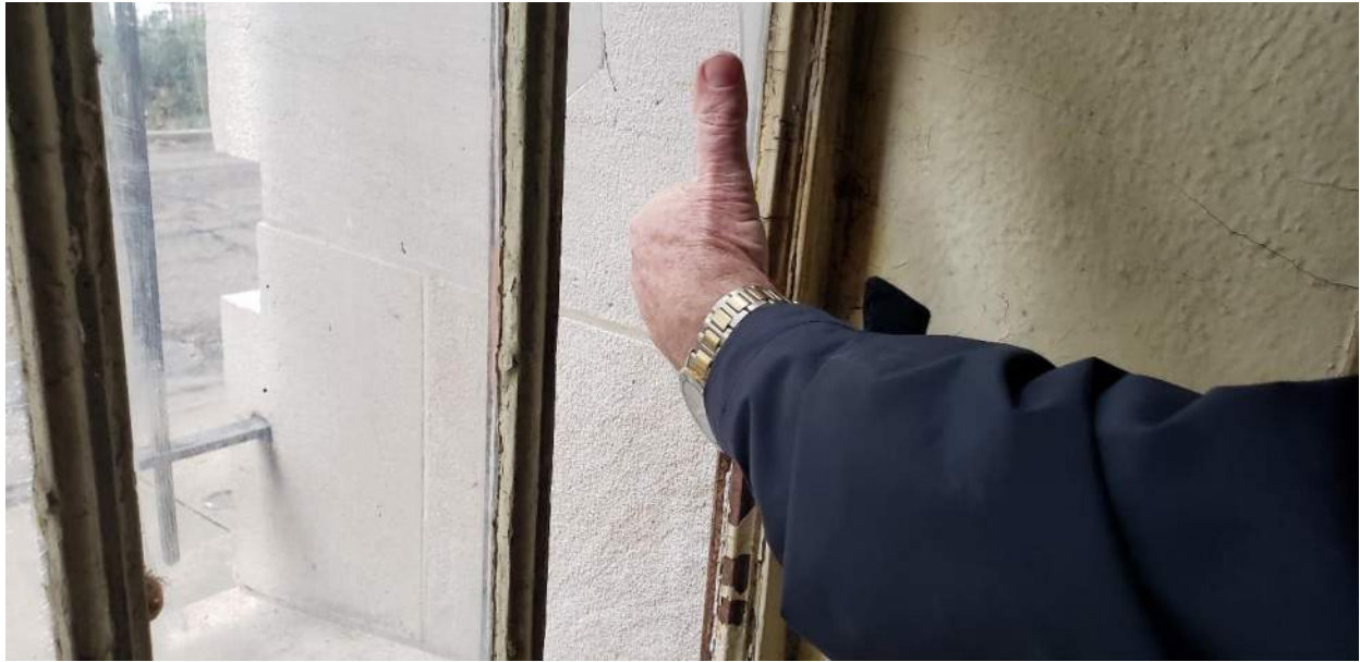
Photo 47: Inside of Window C
