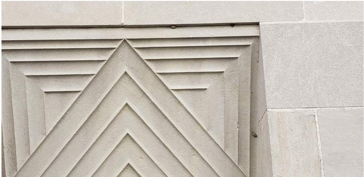
Photo 46: Limestone Header @ Area A @ N. Rampart Elevation
