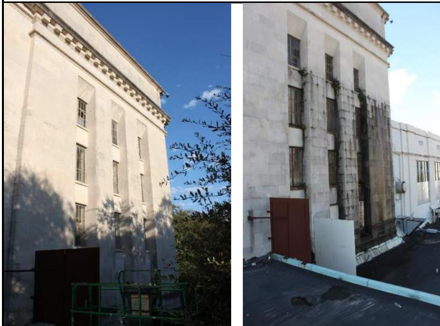
Photo 26: Type C: "Masonry Opng. Steel Casement Opng. Out"
