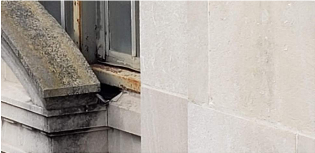
Photo 43: Window A – Lead Flashing
