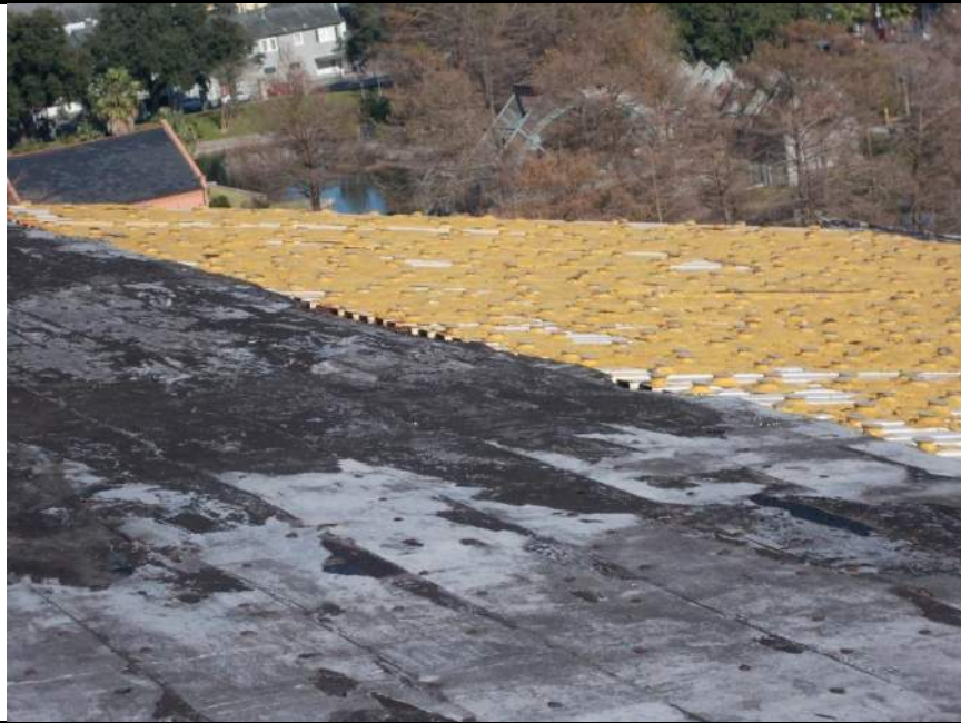
Photo 59: Area of Barrel Vault Covered with Metal Deck.
