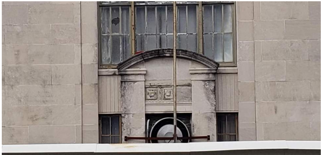
Photo 42: Window A Sill
