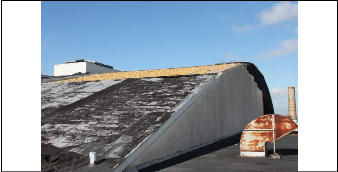
Photo 7: Segmented Barrel Vault Roof with Gabled End
