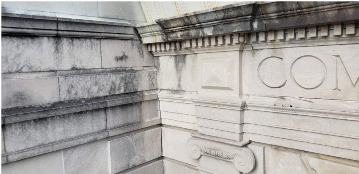
Photo 86: Existing Limestone at N. Rampart Covered Porch
