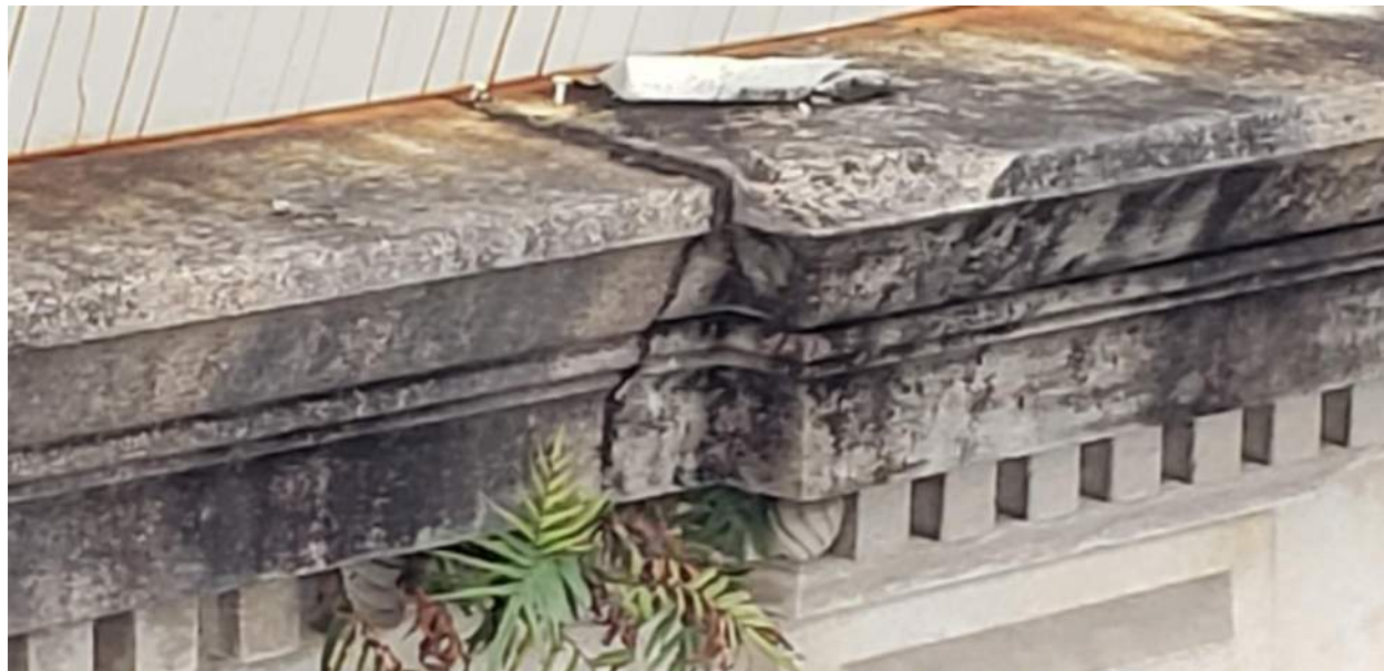
Photo 34: Cornice on Section C (Covered Porch @ N. Rampart)
