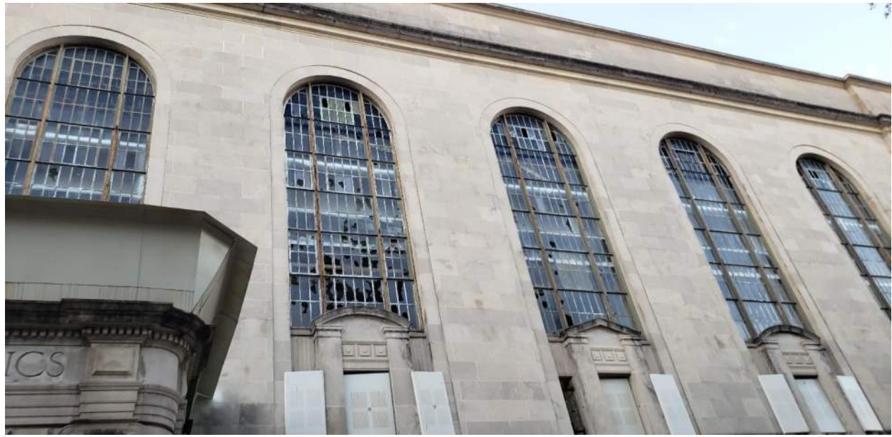
Photo 103: N. Rampart Elevation. Window Type A.
