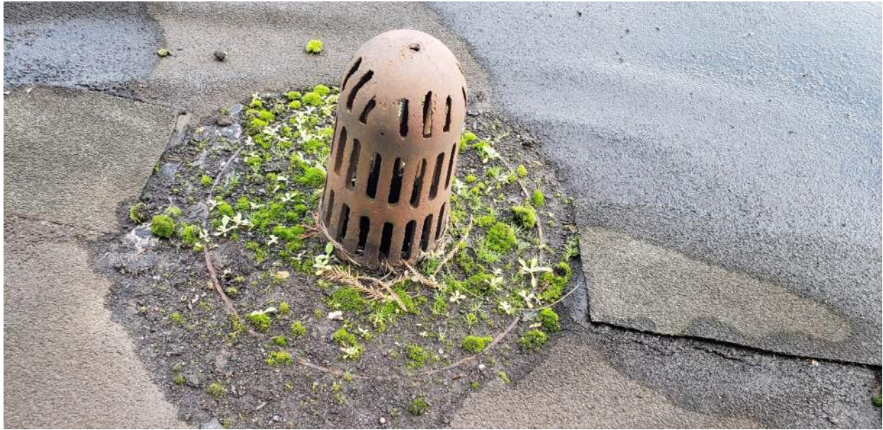
Photo 79: Roof E Area Drain
