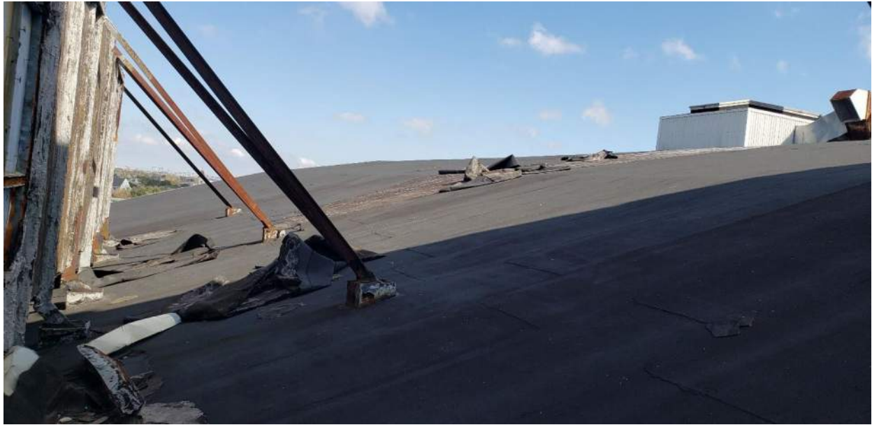
Photo 91: Attachment of HVAC System Housing to Roof.
