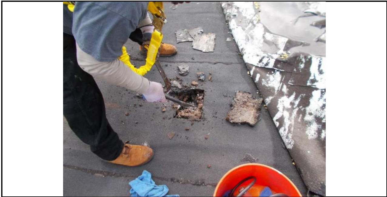
Photo 67: Roof A Core
