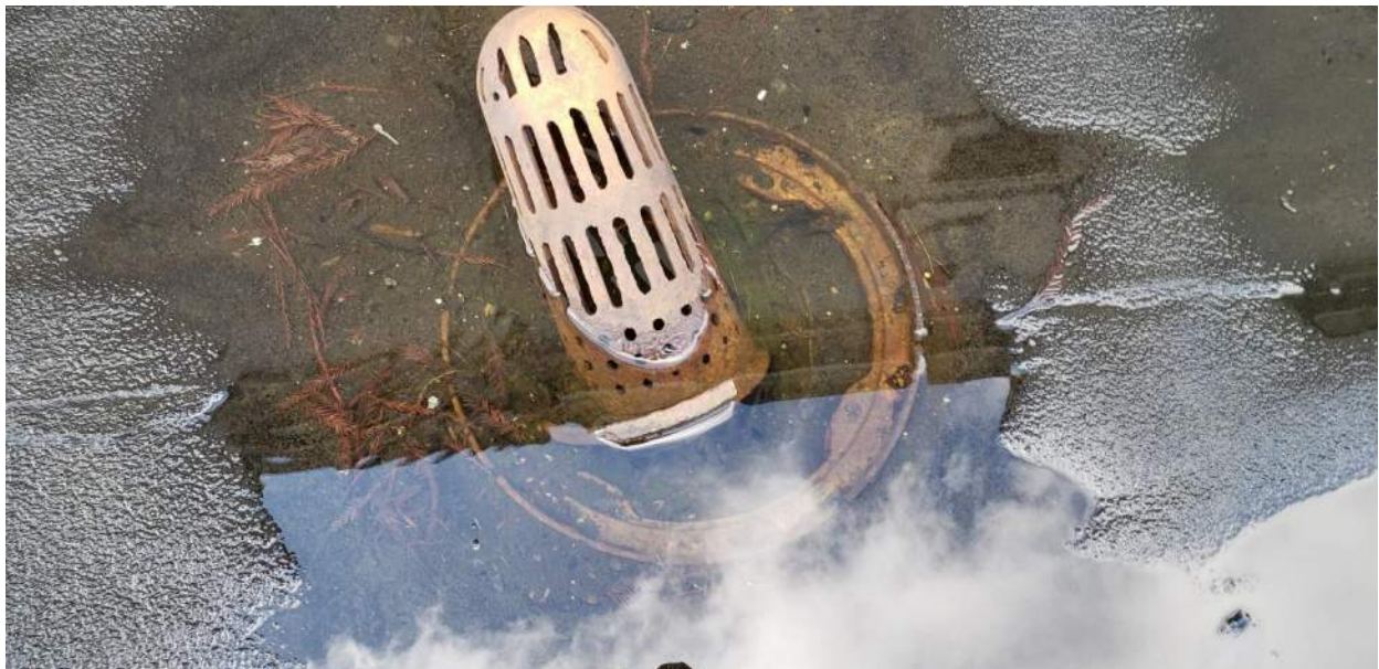
Photo 78: Roof E Area Drain
