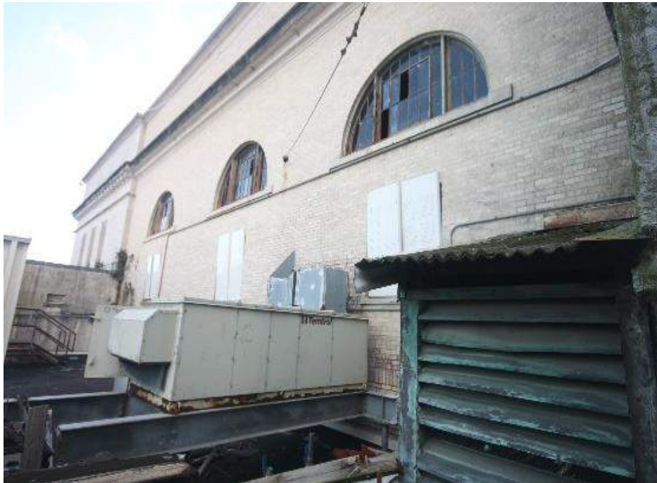
Photo 32: Type K: “Masonry Opening Steel Sash (Projected Type)”
