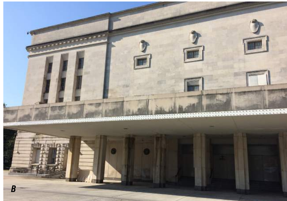
D) SEPTEMBER 2019 PHOTOS OF ANNEX AFTER ALTERATIONS.
