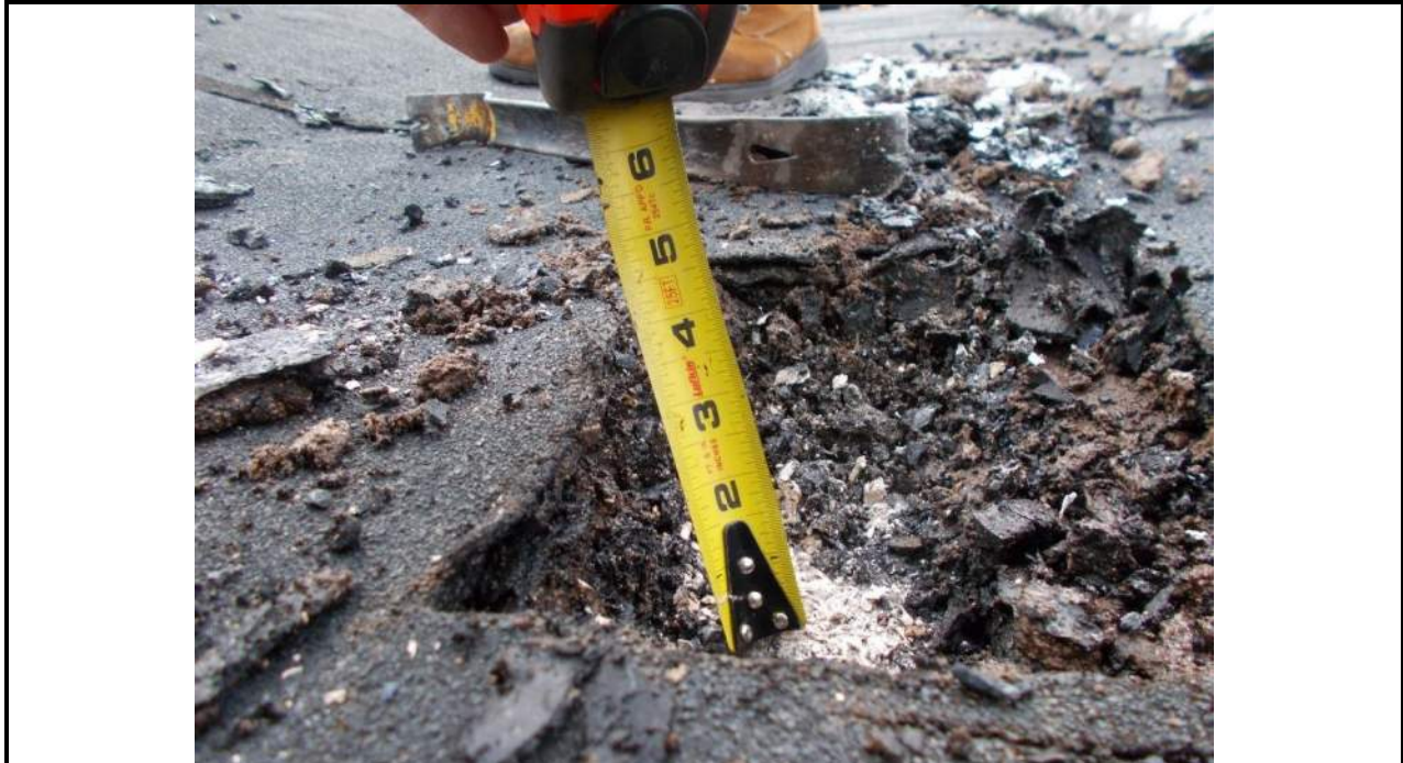
Photo 68: Roof A Core
