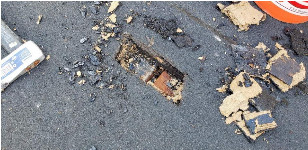
Photo 82: Roof E - Core #2
