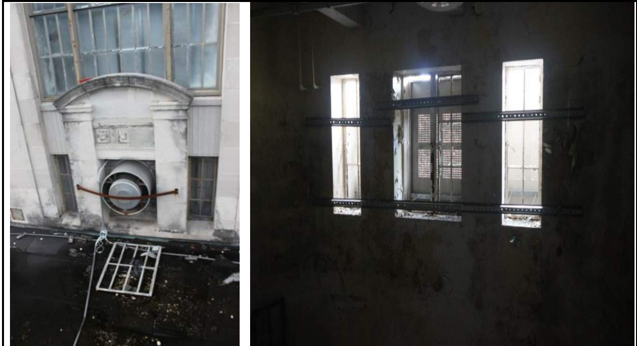
Photo 24: Type F and E “Masonry Opng. Steel Casement Opng. Out”
