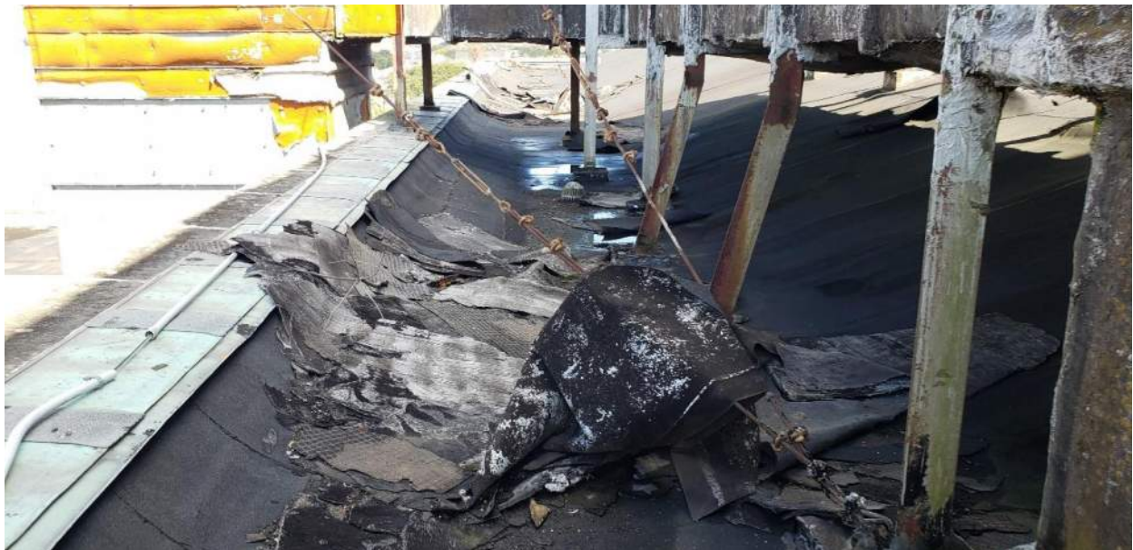
Photo 92: Attachment of HVAC System Housing to Roof.
