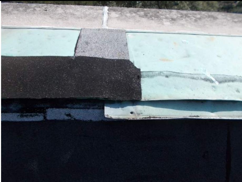
Photo 66: Condition of Base Flashing on Roof A
