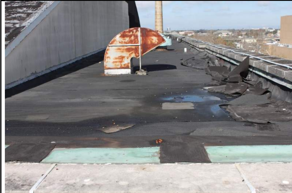
Photo 21: Flat Area of Roof at St. Ann Street Side.
