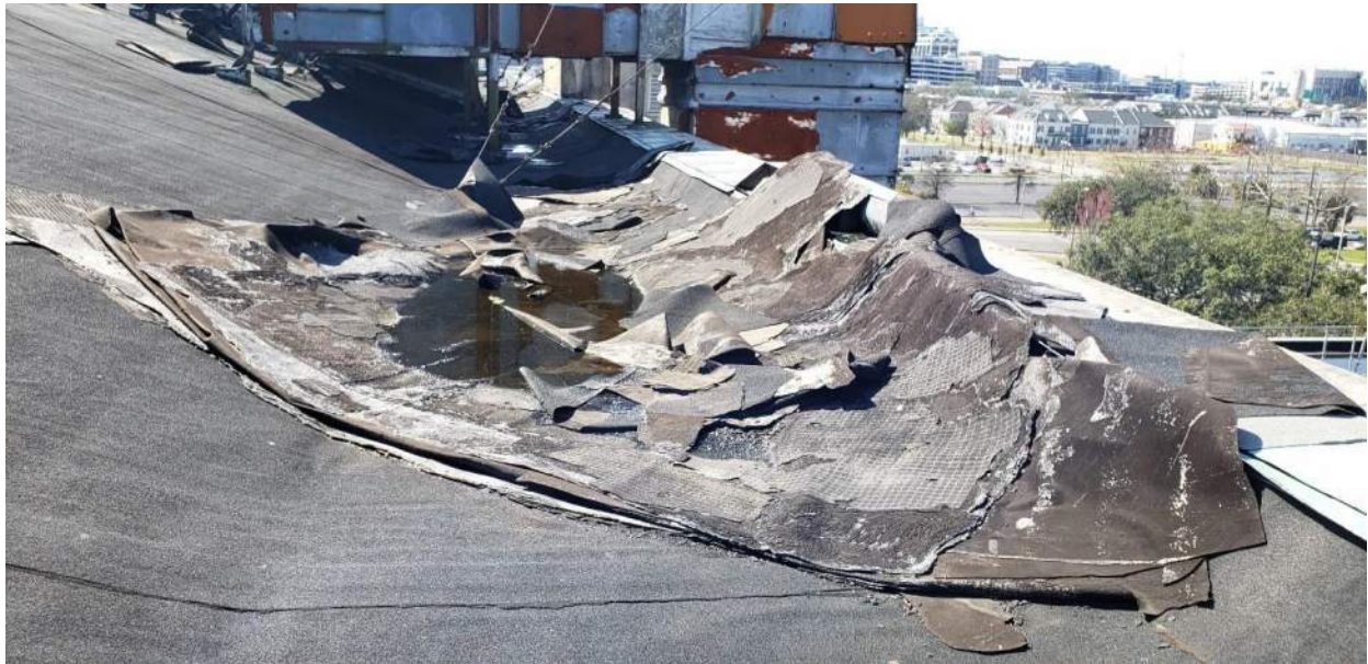
Photo 52: Roof Valley Along Essence Way
