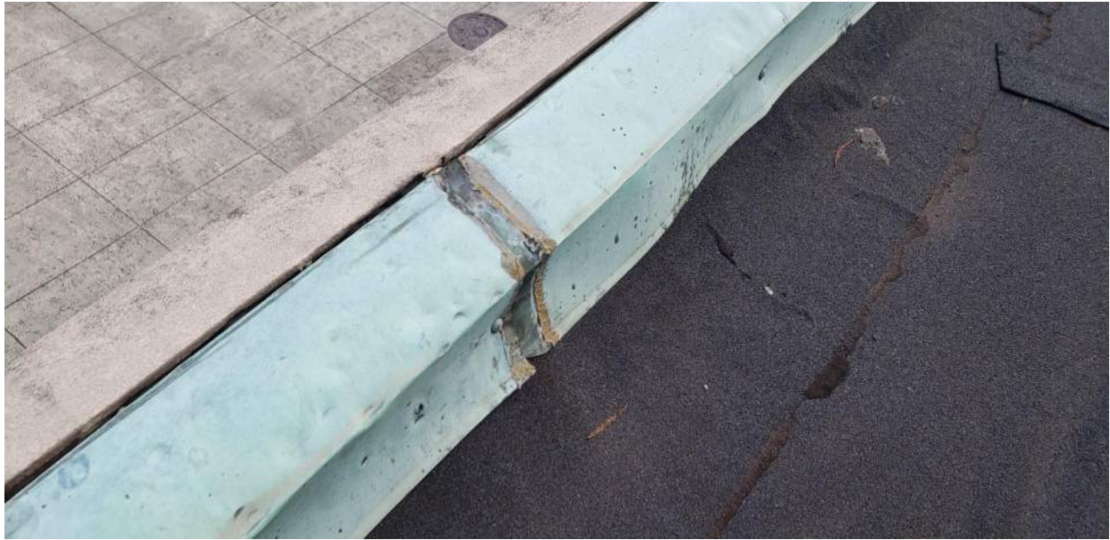
Photo 77: Roof E Coping
