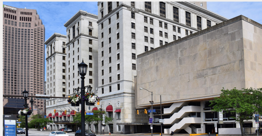
G - W 3rd & Superior facing southeast
