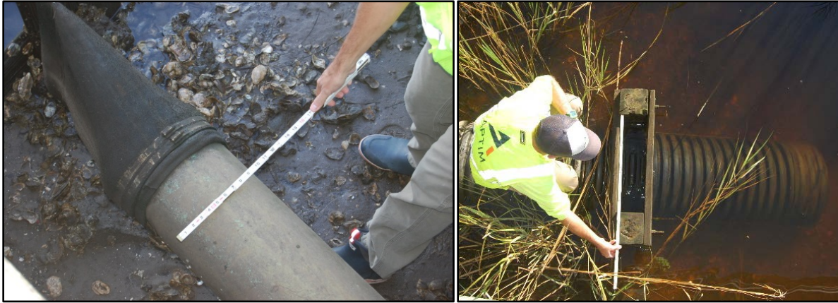
Figure 21. APTIM Conducting Stormwater Outfall Observations.
