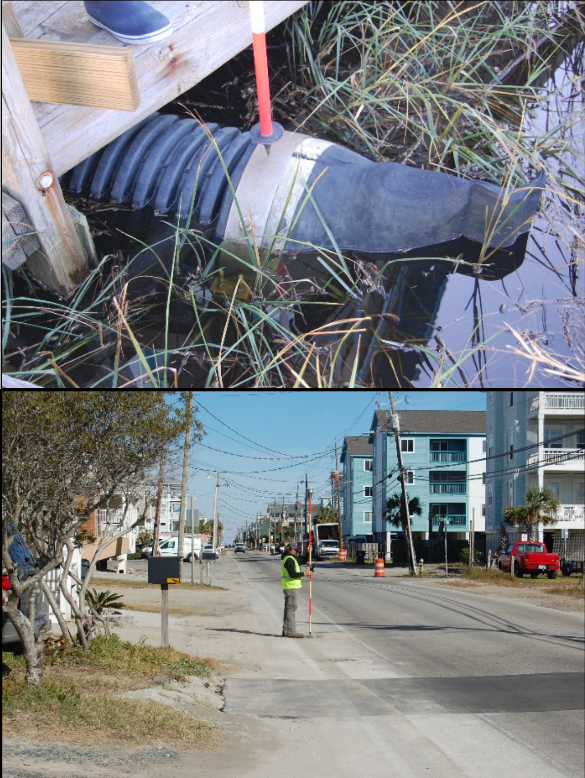
Figure 14. Surveying an Outfall Pipe Located at 909 Canal Drive (upper). Surveying Stormwater Inlets Along Canal Drive (lower).
