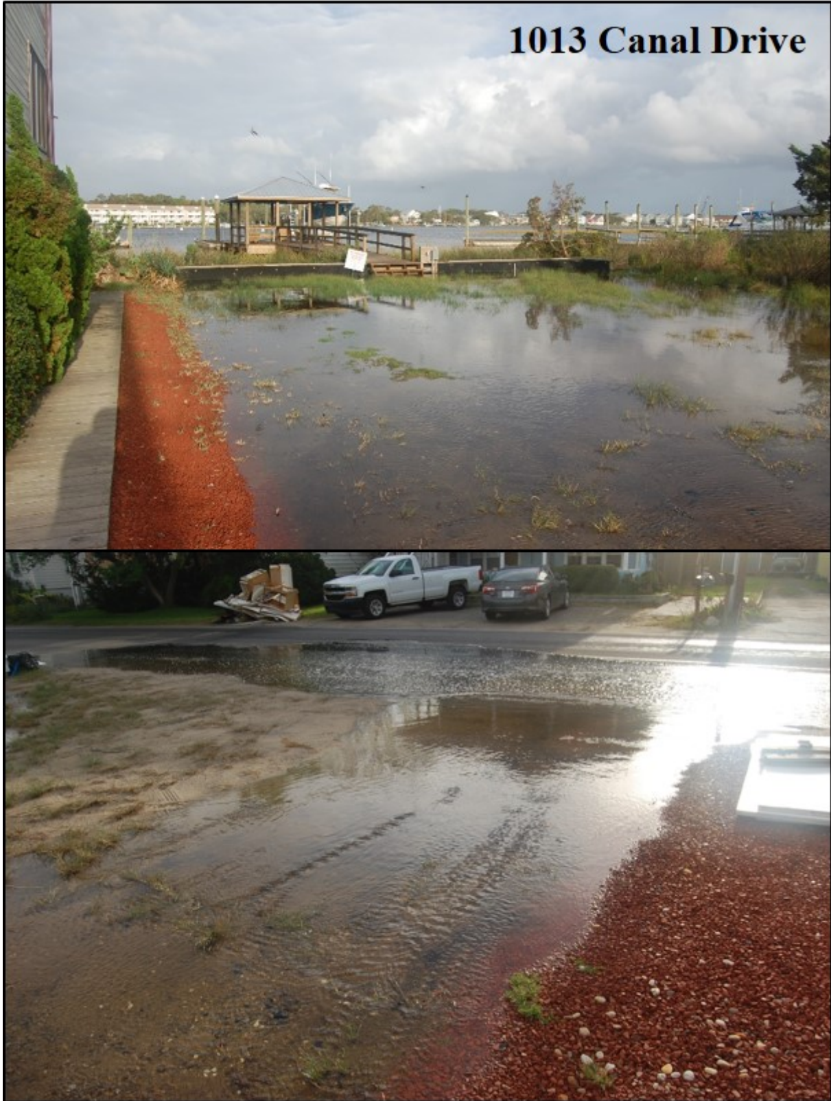
Figure 19. View of high tide flooding around bulkhead at 1013 Canal Drive (upper) and water flowing from the property onto Canal Drive (lower).
