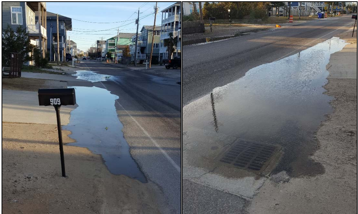
Figure 24. Water Coming Up Through Street Inlets During High Tide at 909 and 911 Canal Drive.
