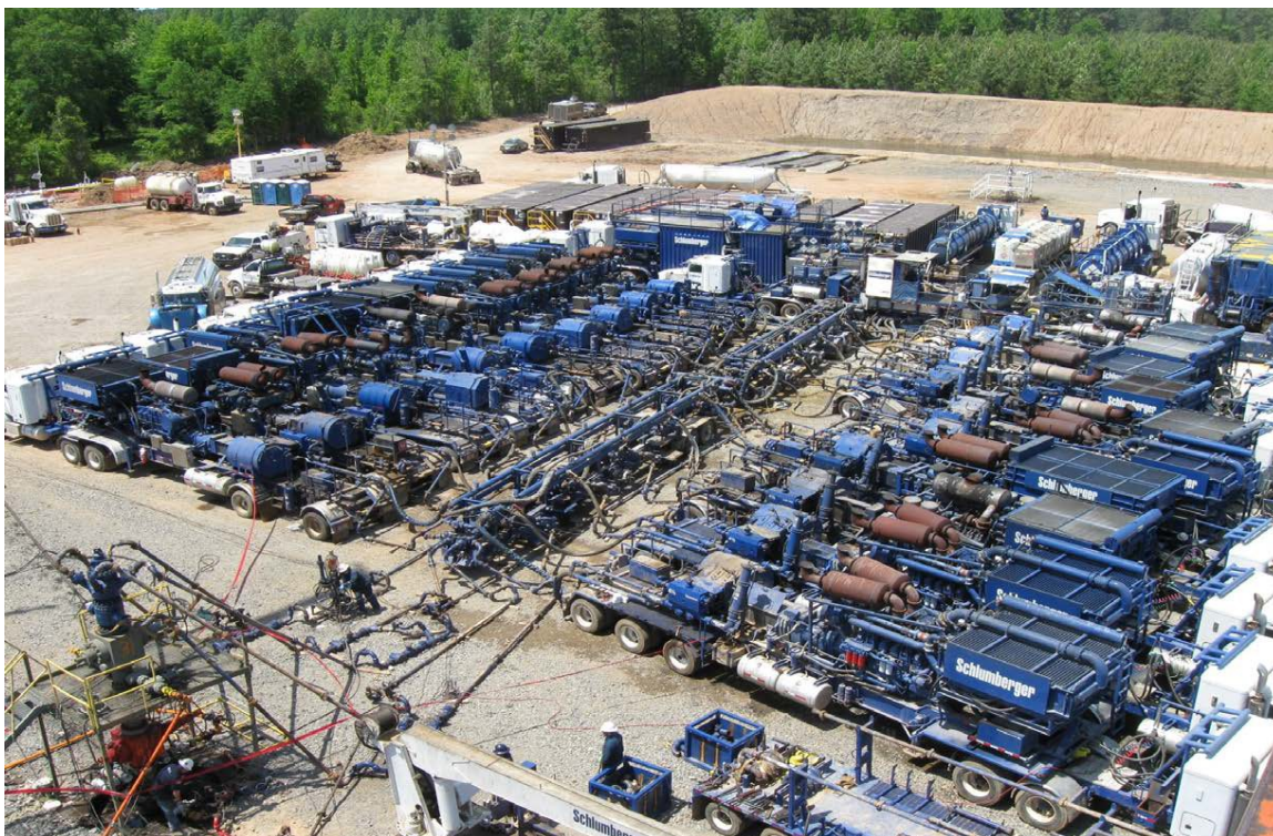
Figure 5-2. Hydraulic fracturing site showing equipment used on-site during the chemical mixing process.
