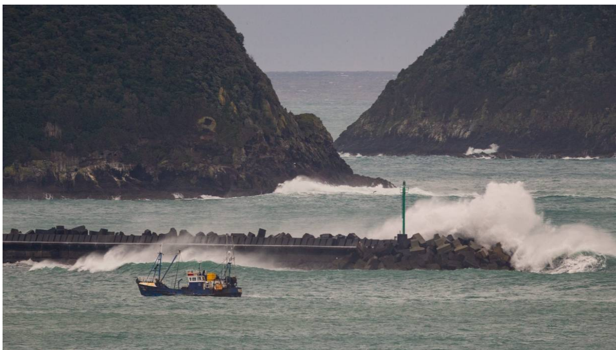
Figure 1: Port Taranaki Main Breakwater
