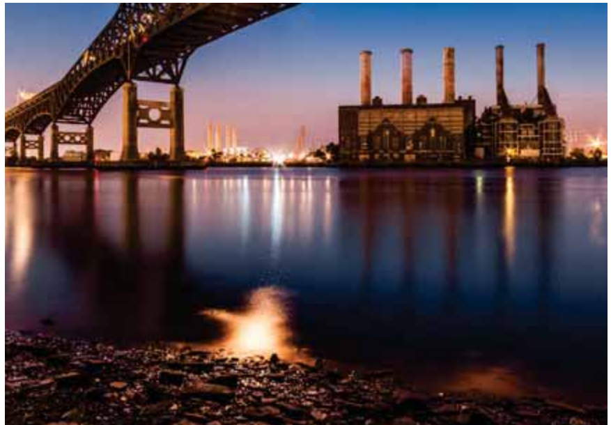
Kearny Power Station, Jersey City, NJ
