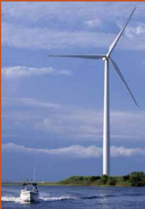
Wind Turbine, Atlantic City, NJ
