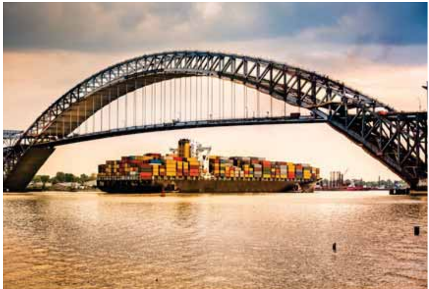
Bayonne Bridge, NJ
