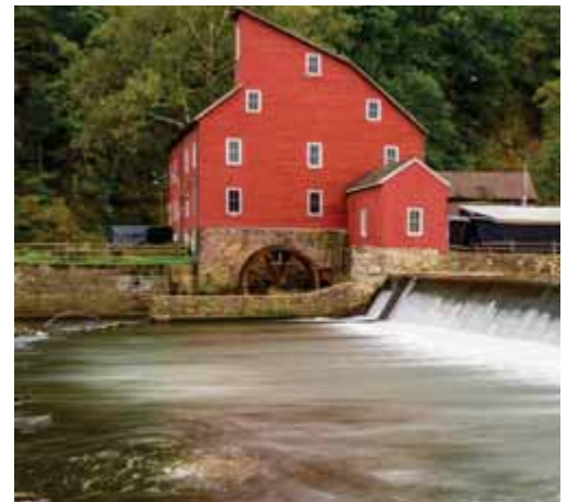
Historic Red Mill, Clinton NJ
