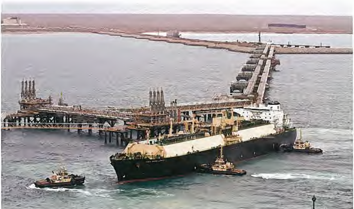
March 2016: Departure of the first LNG cargo on the vessel Asia Excellence. The jetty, loading arms and materials offloading facility can also be seen in this photo..
