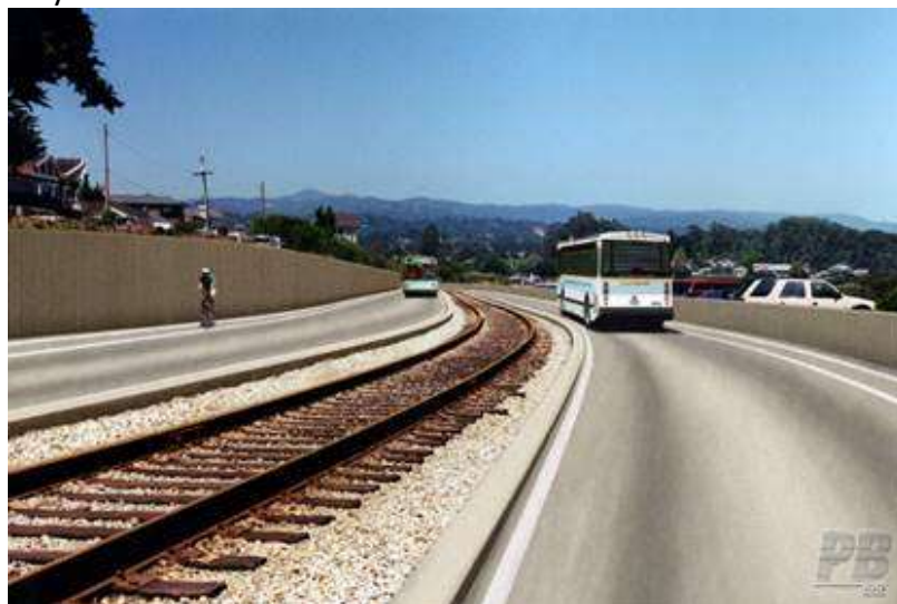
Figure A-1. Photo simulation from MTIS of busway, tracks and bike lanes along the rail right-of-way
