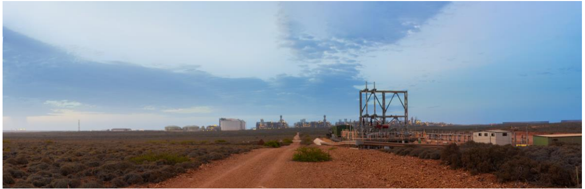
Figure 1 View looking over injection drill centre A showing the manifold and the injection wells (extreme right of image) and the gas processing plant in the background
