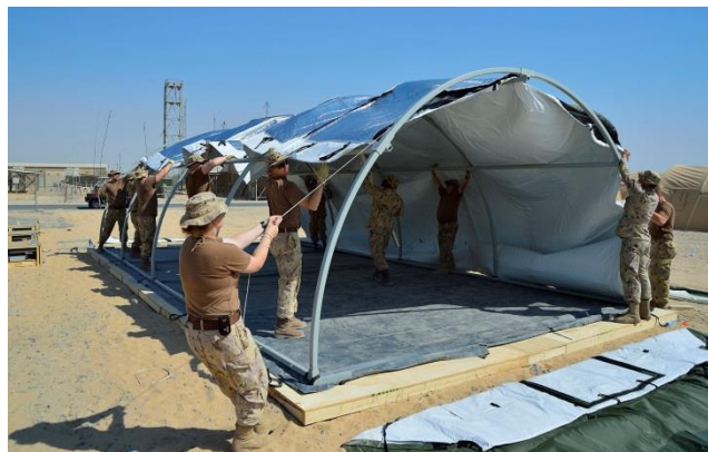
Figure 2-1: Construction of structures in Kuwait
