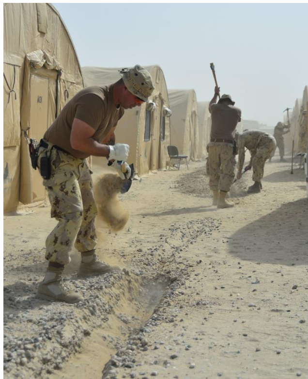
Figure 2-4: Digging trenches for communications conduits
