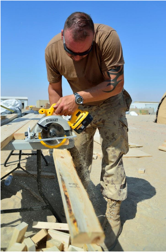
Figure 2-2: Cutting wood to build shelters
