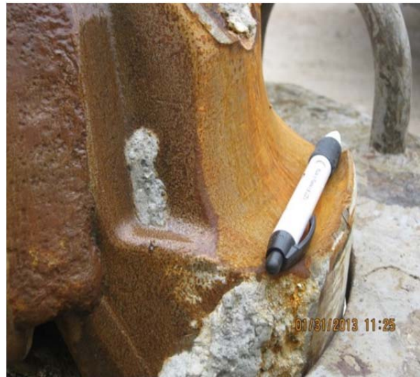
Figure 6: FDEP Photo Indicating Damage to Drill Bit
