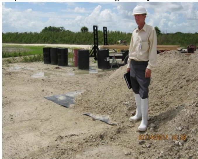
Figure 4: Foreground- What Appears To Be Contaminated Rubble with Improper Containment and Coverage; Background- Barrels of Chemical with No Obvious Secondary Containment
