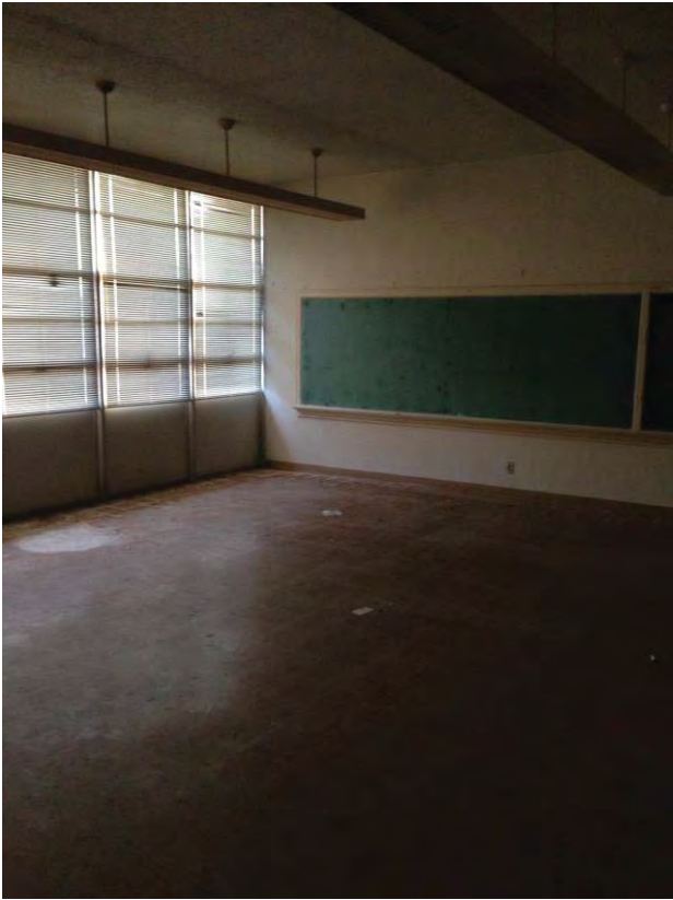
Classroom space with original chalkboards
