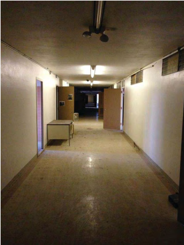
Hallway space, same size upstairs and downstairs
