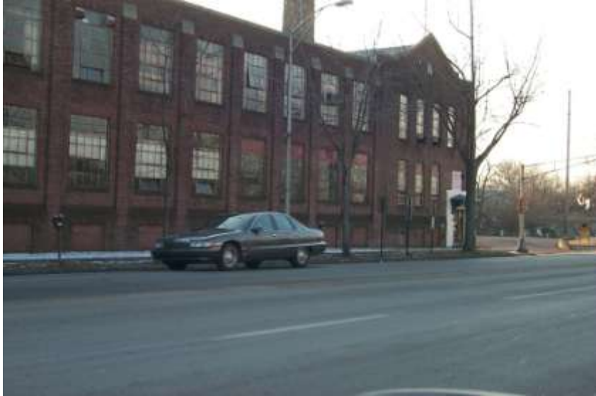
MCCC North Building prior to renovations (Former Nittany Warehouse)
