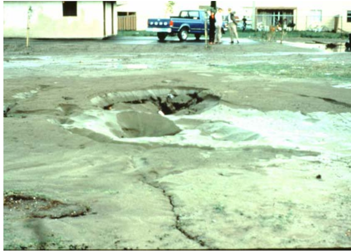
Figure 3.4 Liquefaction on Treasure Island after Loma Prieta Earthquake (TI-HRA-16)
