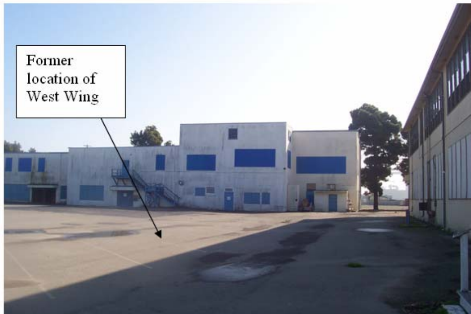
Figure 8.3-14 Former Location of Building 7 West Wing
