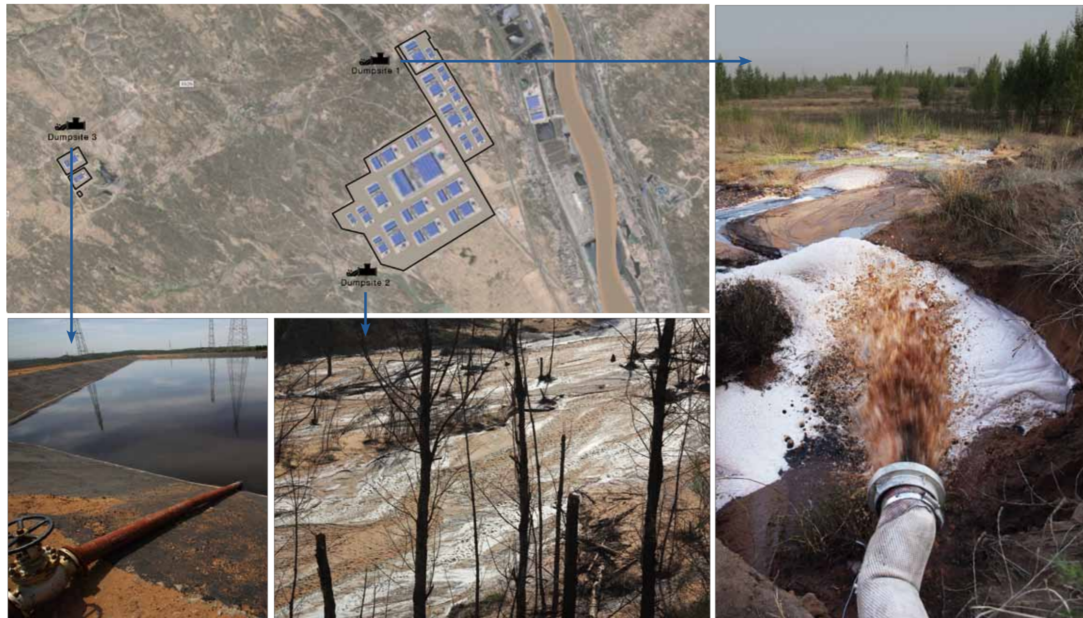
The location of Shenhua's Coal-to-Liquid Project's 3 dumping sites and corresponding on-site photos. ©Greenpeace/Bo Qiu
