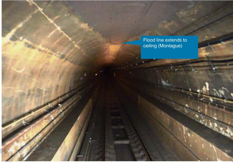
Montague cable replacement work is complicated by damaged concrete and terracotta 'duct banks' that must be demolished and rebuilt
