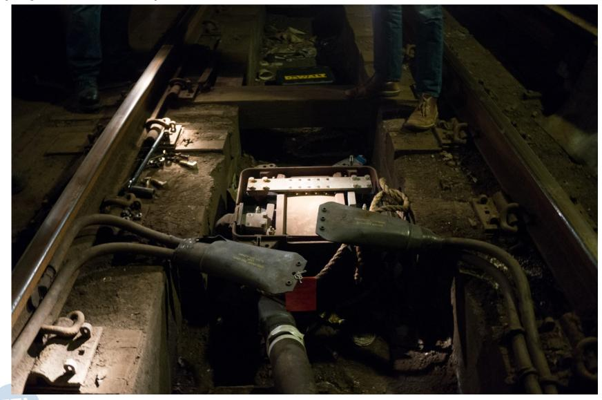
Montague and Greenpoint tube damage – circuit breaker house damage that could reduce power reliability
