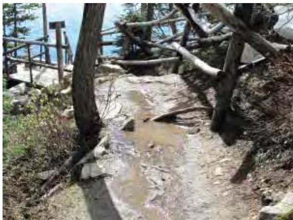
Trail conditions near the west boat launch
