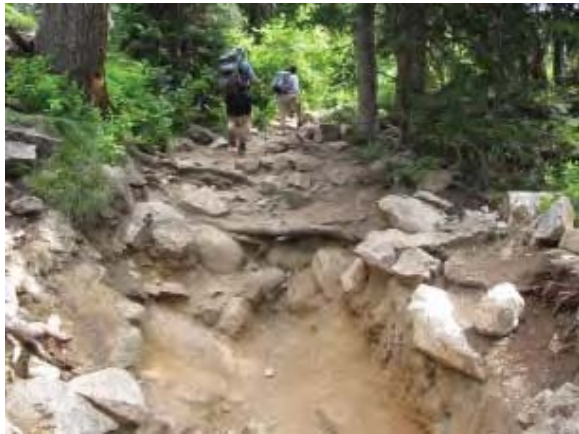
Rugged trail conditions on the way to Hidden Falls/ Inspiration Point caused by erosion
