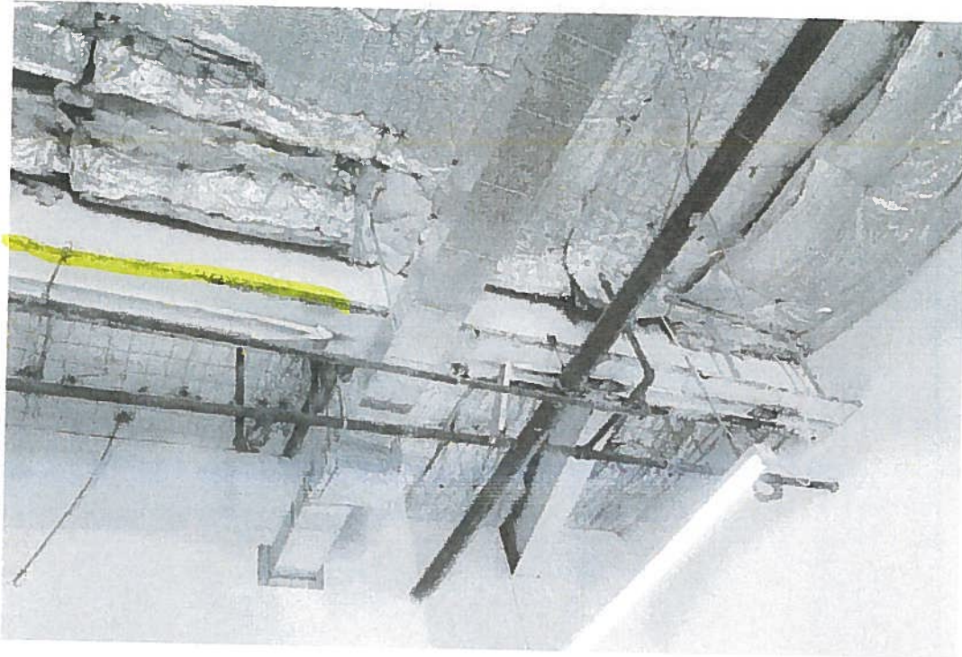
Picture 7: Rusting on steel beams in receiving of Zellers.
