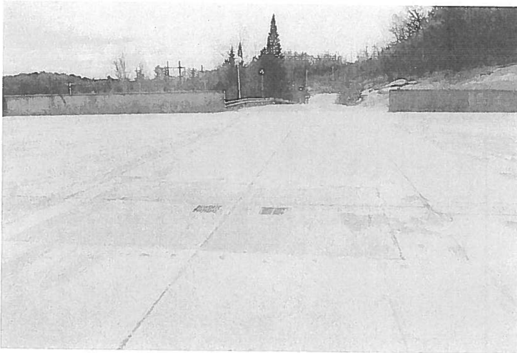
Picture 2: South entry to parking deck above Zellers..
